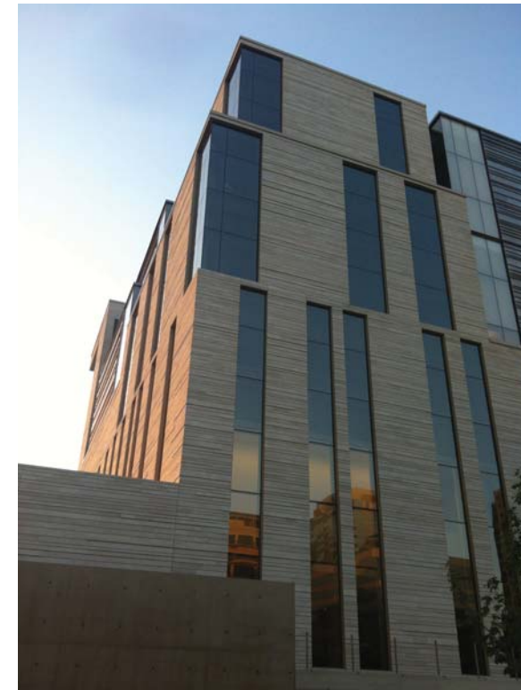
Comments from the Downtown Design Commission indicate a preference for a structure that meets the 21st century appeal of the new Federal Courthouse building.
