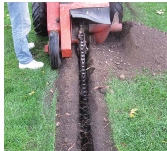
Root pruning can be done as a preventative measure before starting invasive excavations.
