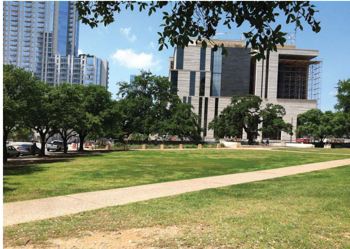
Views to the west are dominated by the new Austin Federal Courthouse, "Auction Oaks," and wood deck area recently added to the Park. (Photo by Design Workshop)
