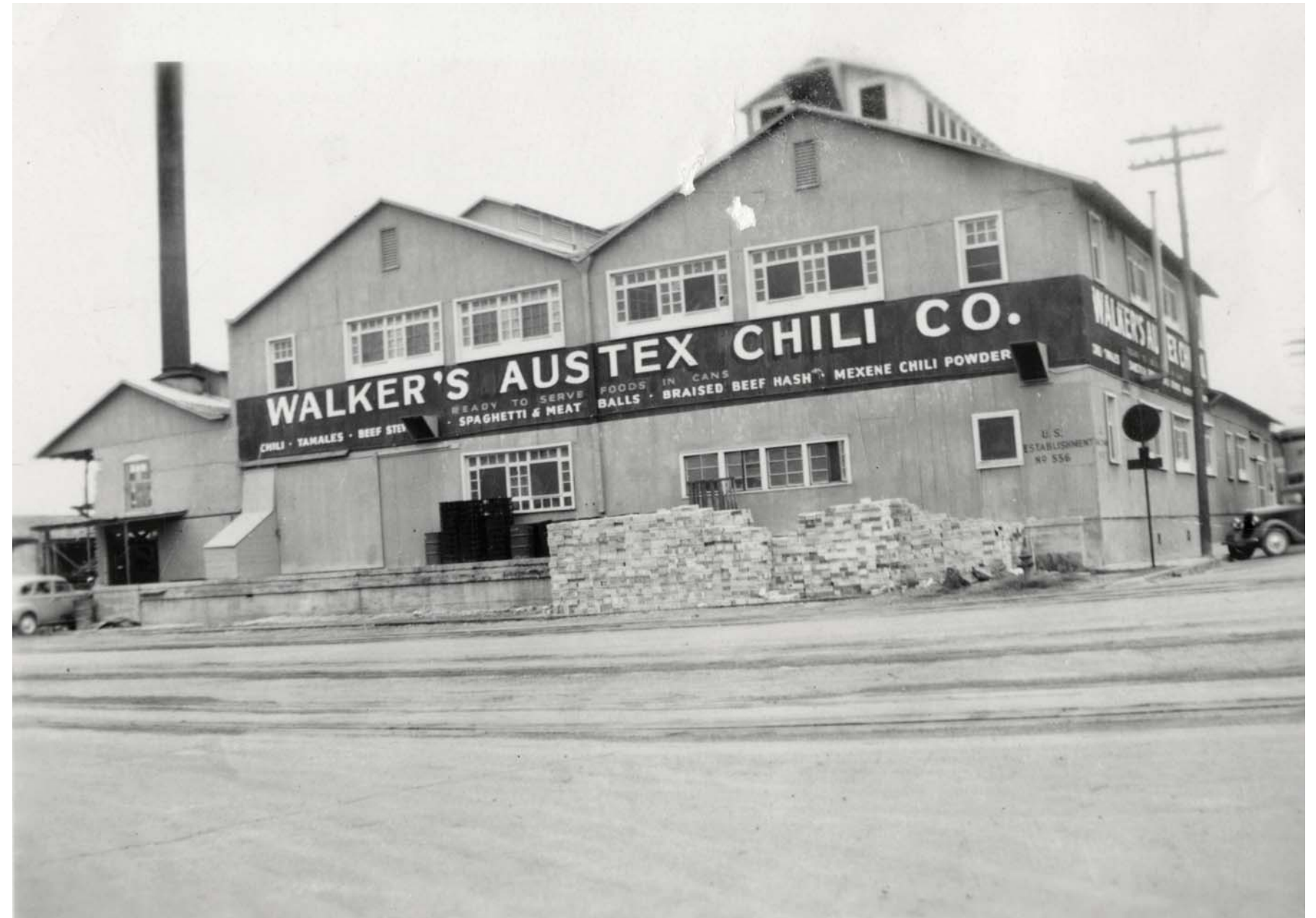
Walker's Austex Chili Factory was found in 1900 located one block south of the Park and employed approximately 15% of the city's Mexican and Mexican-American population. After a fire in 1916, the factory was rebuilt one block west (PICA 15019, Austin History Center, Austin Public Library).
