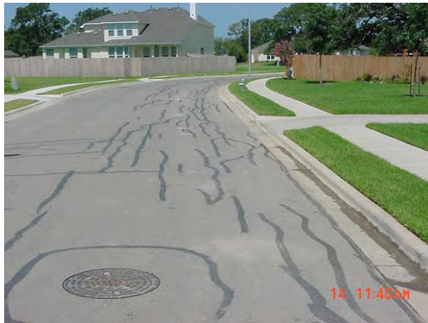
Left: Photo of pavement cracks in a new Austin subdivision in 2009. Right: Longitudinal cracking on Golden Falls Drive in Travis County in 2008. Photo credit: City of Austin.
