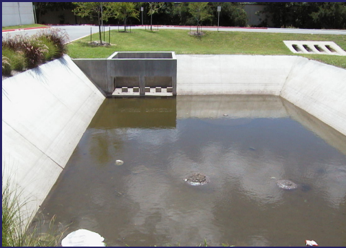
Example: Stormwater Ponds
