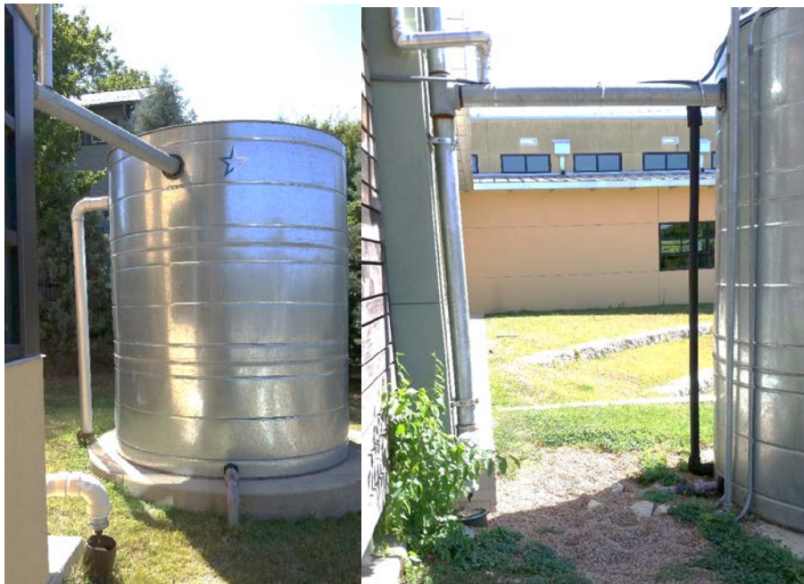
Photos showing connection to roof downspout and outflow to below-ground irrigation system.
