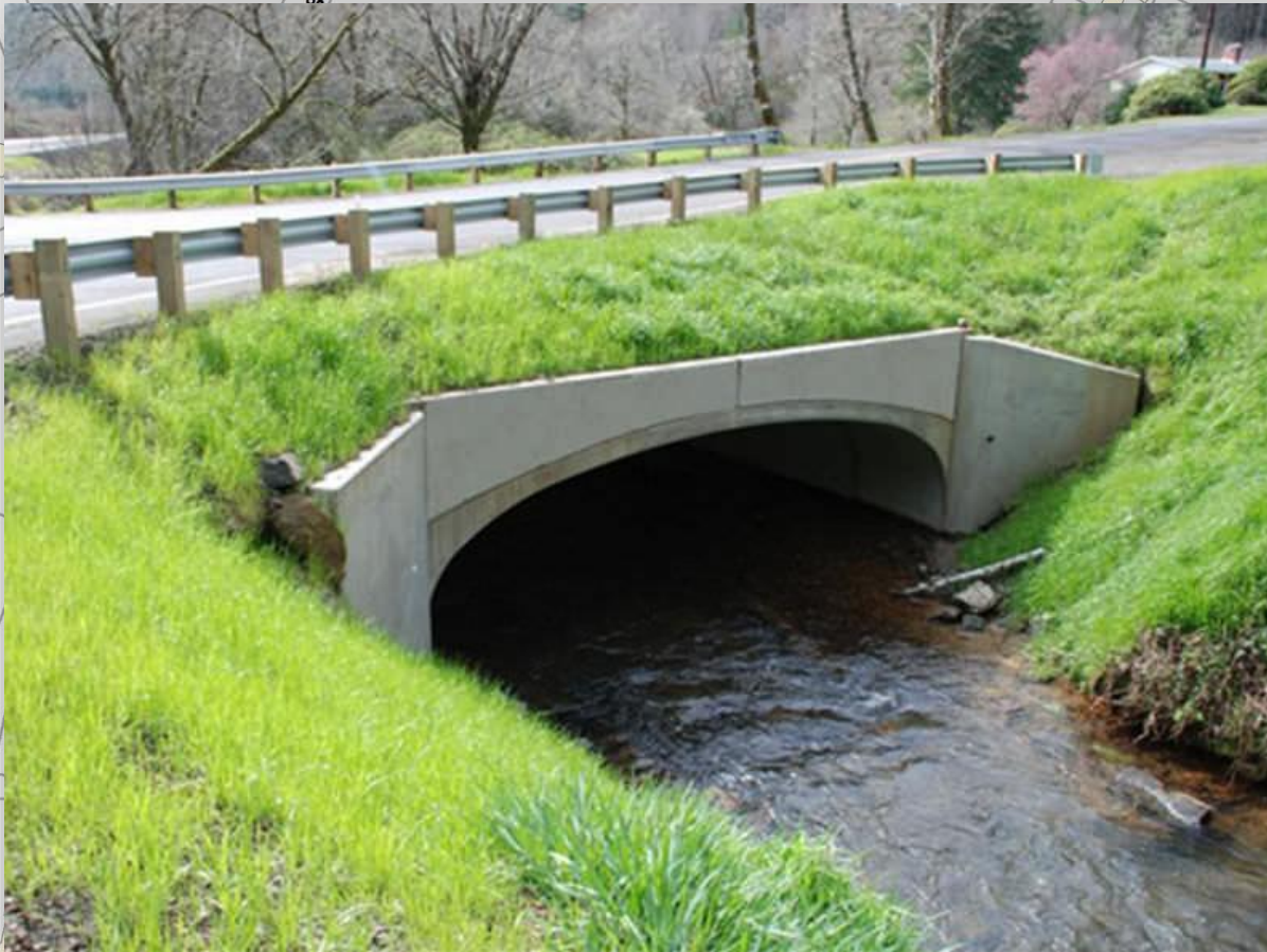
Existing Stormdrain System
