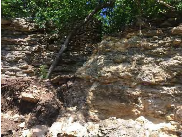
Upslope edge of failure at 2431 Wooldridge Drive Mortared natural ledge stone landscape wall Looking west near north end of failure
