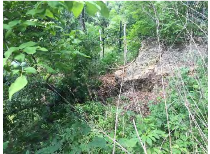
Near NW corner of fence for 2431 Wooldridge Drive locally displaced Near downslope and northern edge of slide
