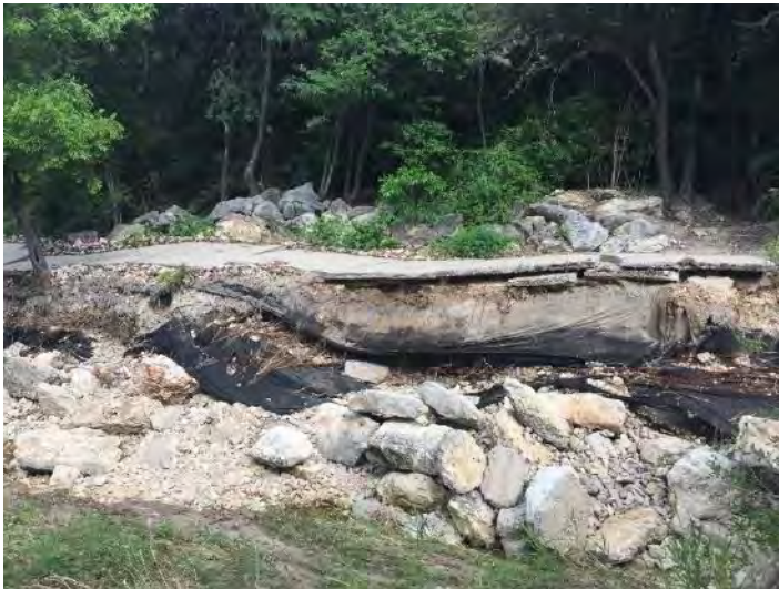
D/S half of horiz. trail wall displacement at Shoal Creek Creek bed material pushed up into pile in front of slide Displacement greater in downstream (d/s) half compared to upstream (u/s) half
