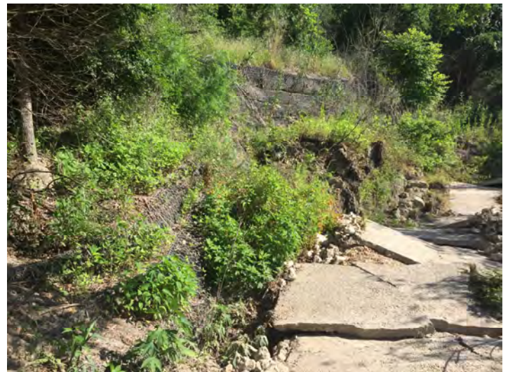
Existing gabion wall Note bulging displaced gabion toe at south end and heaving/thrusting of material at front face
