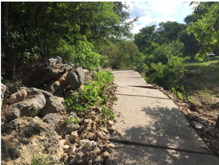
Along trail south of existing gabion wall Some vertical displacement of pavement, mostly horizontal
