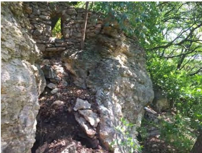
North edge 2431 Wooldridge Drive Potential older failure - parallel to new failure Location of misc. natural ledge stone walls Looking north
