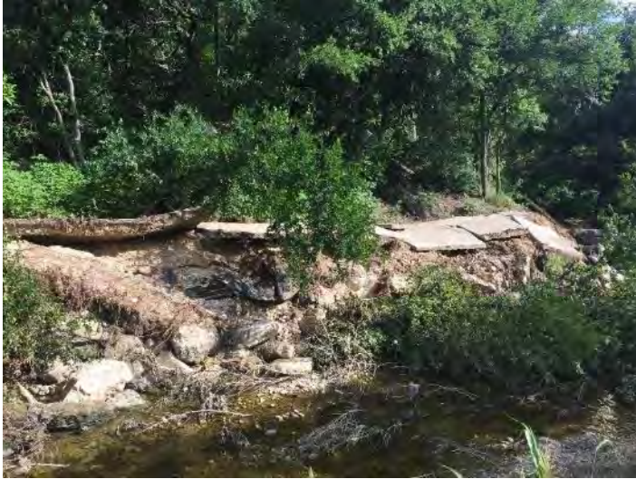
Upstream (u/s) half of horiz. trail wall displacement at Shoal Creek Displacement of bed material not as significant
