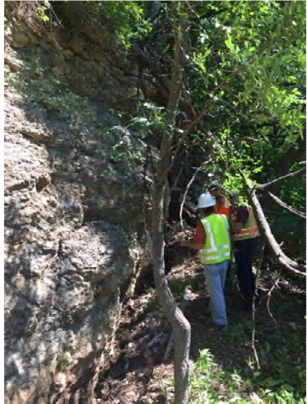
Older failure along north edge of 2431 Wooldridge Drive Soil on right and Buda rock face on left (looking north). Note slight separation at base parallel to new failure
