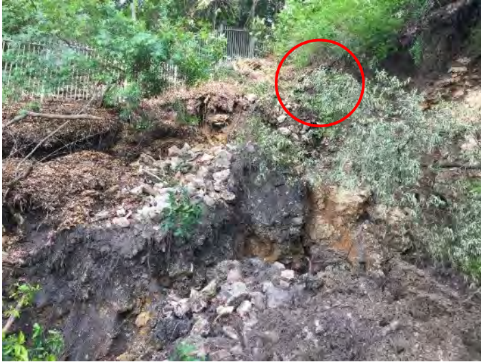
Southern edge of slope failure along fence line at 2419 Wooldridge Drive Deep crevasse and separation along fence line. Upper right hand corner – existing storm drain
