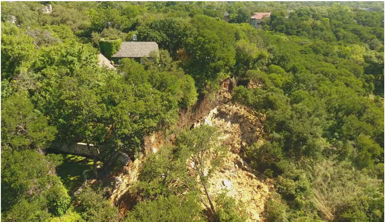
Looking north along 2421 and 2431 Wooldridge Drive (drone video from City)
