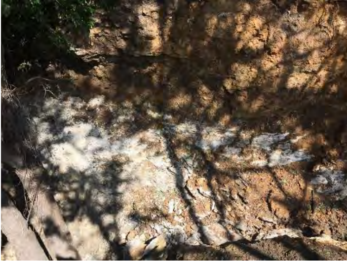
Close up of Buda/Del Rio contact location Along south end of 2431 Wooldridge Drive
