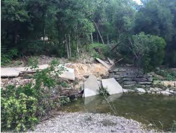
Northern terminus of slide at Shoal Creek Existing dry stack wall pushed horizontally into creek
