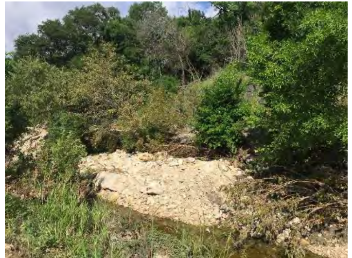
D/S half of horiz. trail wall displacement at Shoal Creek Creek bed material pushed up into pile in front of slide Displacement greater in d/s half compared to u/s half
