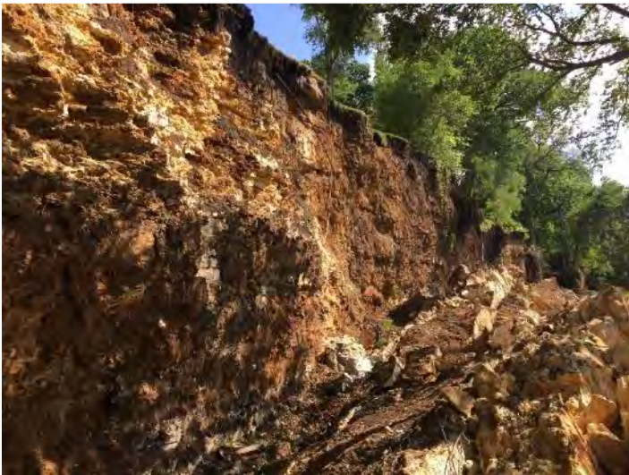
Upslope edge of failure at 2431 Wooldridge Drive Looking north. Unstable slope.
