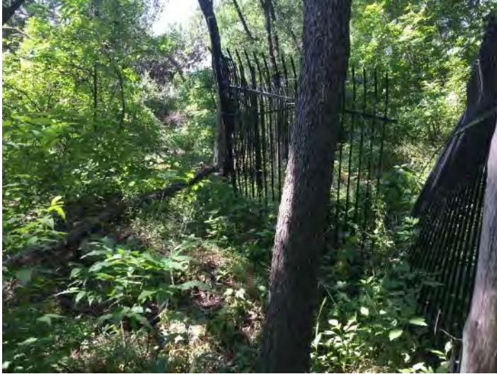
NW corner of fence for 2431 Wooldridge Drive locally displaced Near downslope and northern edge of slide
