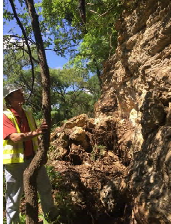
North end of upslope edge of failure at 2431 Wooldridge Drive Buda formation above
