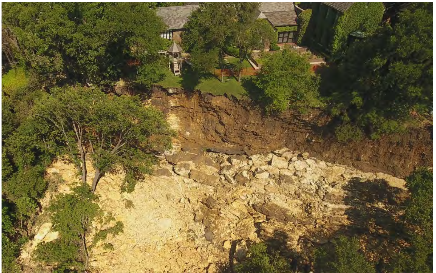
Looking west at 2431 Wooldridge Drive (drone video from City)
