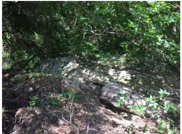
At base of upslope edge of failure at 2431 Wooldridge Drive Landscape wall fallen from yard above
