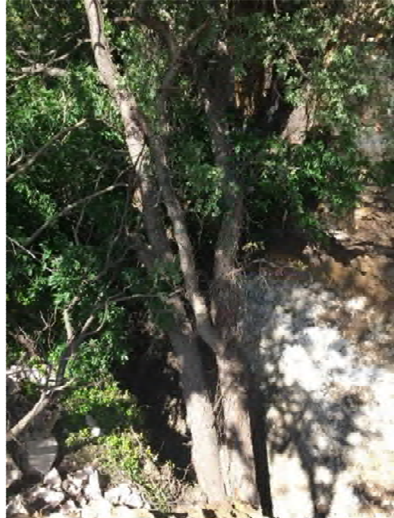
Upslope edge of failure at between 2421 and 2431 Wooldridge Drive Buda Formation (above) Del Rio (below) – contact Note deep separation crevasse behind tree at bottom of pic
