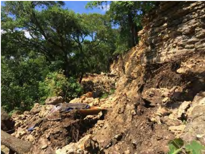
Upslope edge of failure at 2431 Wooldridge Drive Looking south near north end of failure. Unstable slope. Mortared natural ledge stone landscape wall at upper right corner
