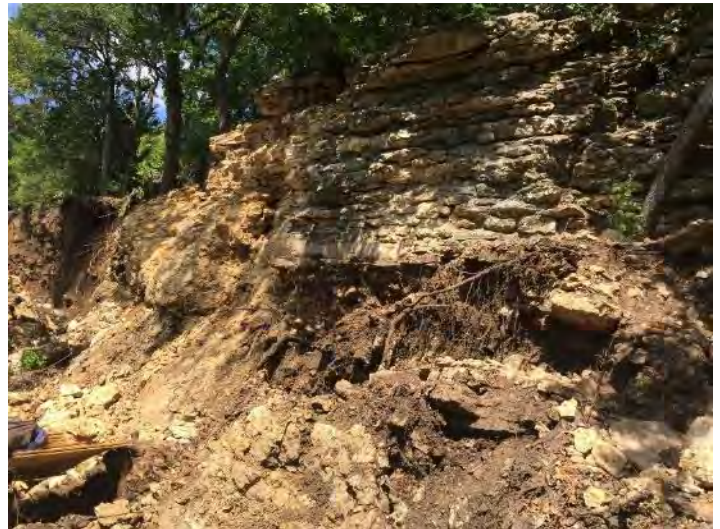
Upslope edge of failure at 2431 Wooldridge Drive Mortared natural ledge stone landscape wall
