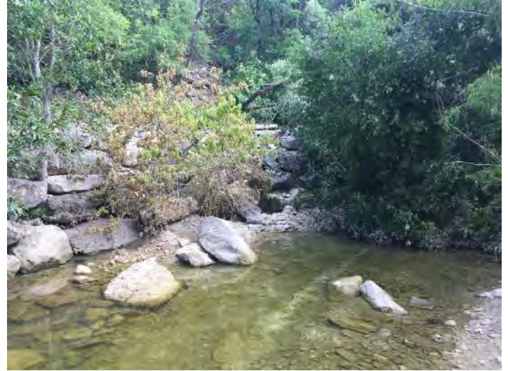
Southern terminus of slide at Shoal Creek Existing dry stack wall pushed horizontally into creek
