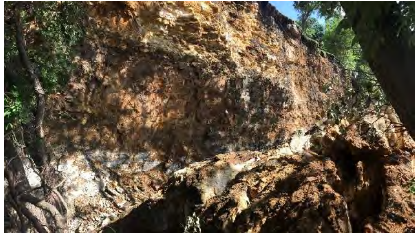
Upslope edge of failure at between 2421 and 2431 Wooldridge Drive Buda Formation (above) Del Rio (below) – contact location Thickness of Buda approx. 20ft. Unstable slope.ft
