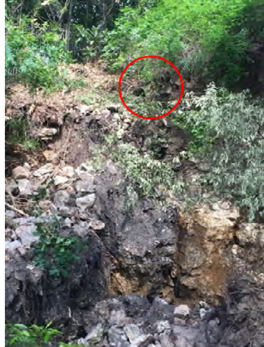
Southern edge of slope failure along fence line Upper right hand corner – existing storm drain
