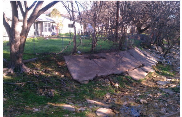
Localized flooding in the Blarwood neighborhood and erosion in the Cherry Creek channel before project construction
