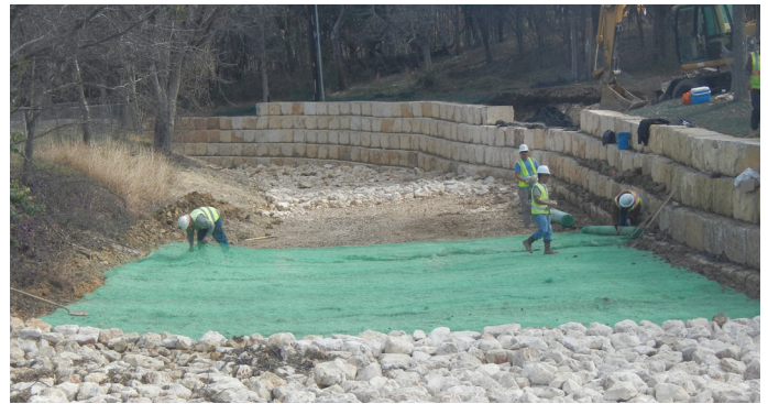
Cherry Creek channel capacity was increased from Blarwood Drive to Coatbridge Drive to offset increases in storm-water flow from the new storm drain system to protect downstream properties and structures.
