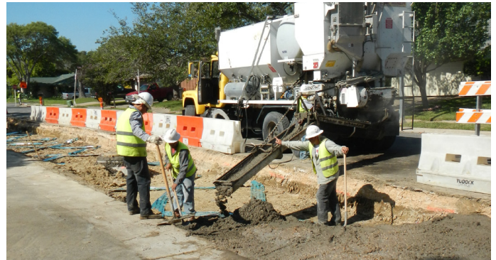
New reinforced concrete pipe and street resurfacing in the Blarwood neighborhood
