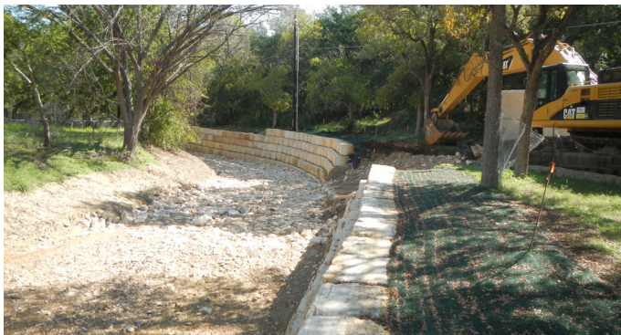
Cherry Creek channel capacity was increased from Blarwood Drive to Coatbridge Drive to offset increases in storm-water flow from the new storm drain system to protect downstream properties and structures.
