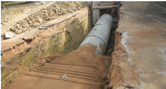
New reinforced concrete pipe and street resurfacing in the Blarwood neighborhood
