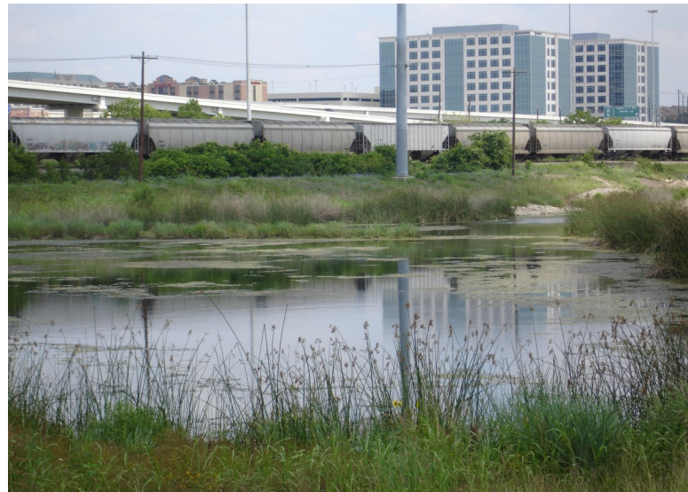
Photo of the Upper Shoal regional water quality and flood detention pond in the Shoal Creek watershed.
