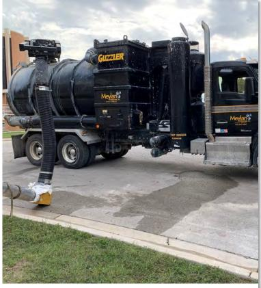
The water and scale residue are then vacuumed from the bottom of the basin using a truck-mounted vacuum
