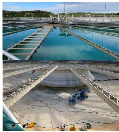
Water is sprayed at high pressure to remove lime scale from basin surfaces
