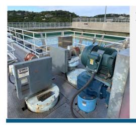
Small motors are used for mixing and stirring of basins and for pumps
