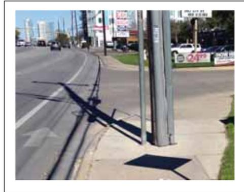
Where sidewalks are present, widths range from 4-feet to 6-feet and are generally directly adjacent to the roadway on the west side and separated by a grassy median on the east side of South Lamar Boulevard. In several locations, utility poles located in the middle of the sidewalk or missing ADA ramps cause accessibility issues. In areas where new development has occurred, sidewalks are even wider and setback from the roadway with a landscaped buffer.
