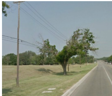
FIGURE 18 — Pruned Tree in FM 969 Right-of- Way
