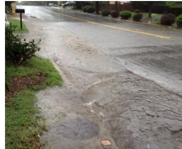
Image of an inlet (foreground) exceeding its capacity and overflow in the gutter.
