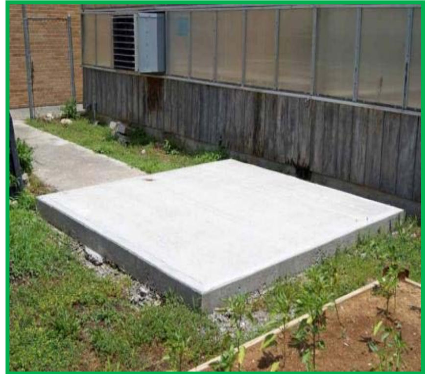
The concrete slab where the rainwater cistern will be installed this fall.
