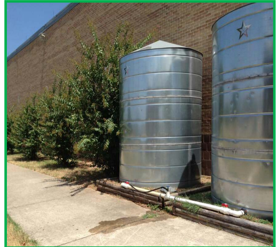
Rainwater collection tanks will help alleviate local flooding issues.
