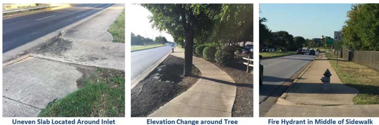
Figure 3-22: Examples of Existing Sidewalk Issues
