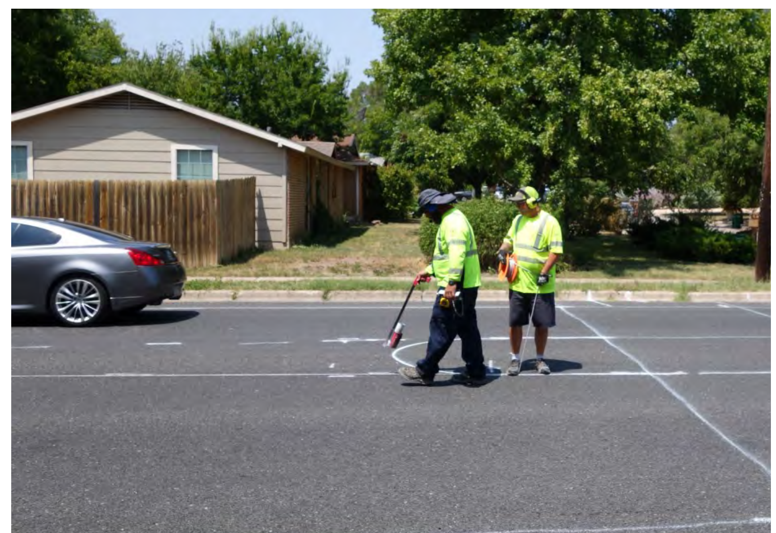
Laying out lines to be striped on Berkman Drive
