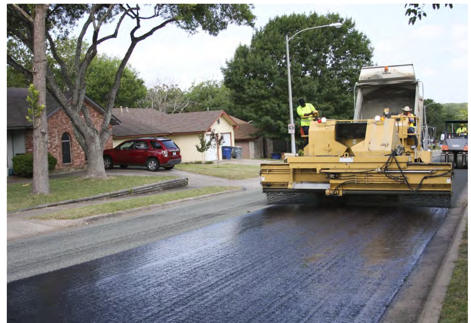
Seal coat resurfacing on a residential street
