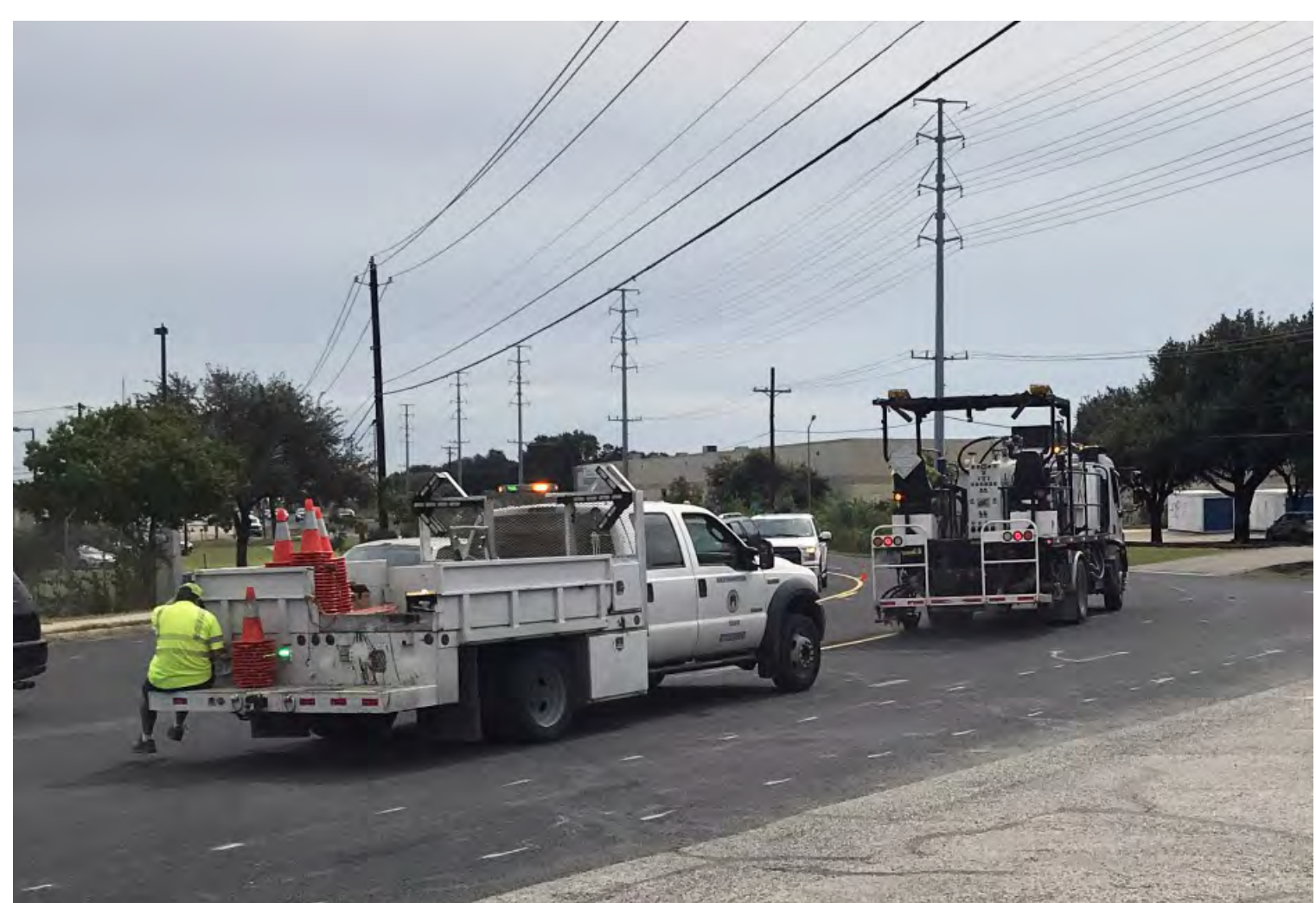
The striping truck painting lines on Burleson Road
