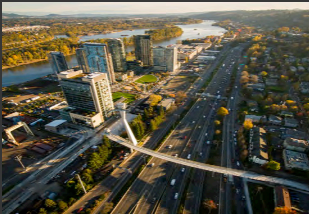
Pedestrian Bridge, South Waterfront
