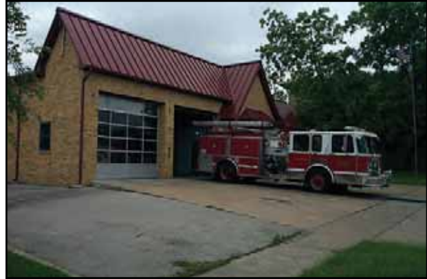
City of Austin fire station
