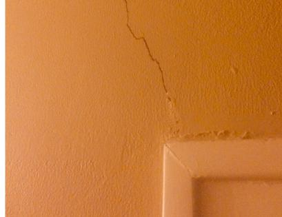
**Above left:** Parts of Austin have clay soils that move based on varying moisture conditions, and early slabs were not always properly reinforced. As a result, many historic slab-ongrade foundations have cracks as a result of settling.
