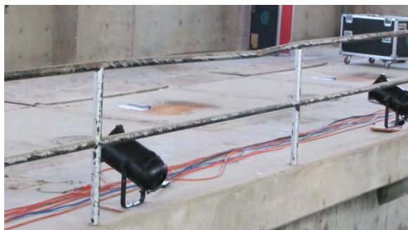
Figure 10. Damage to handrail at Building A
