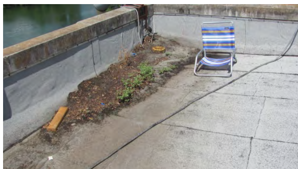
Figure 12. Clogged roof drain at Building A
