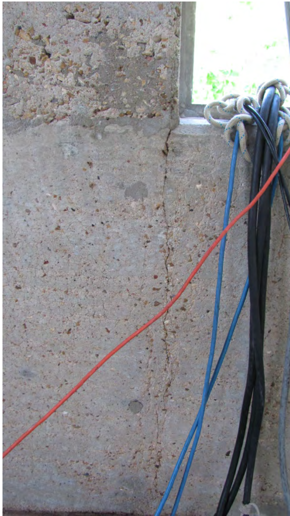
Figure 6. Vertical crack at window in Building A
