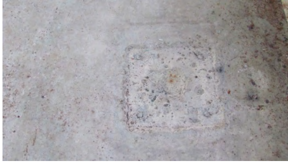
Figure 5. Remnants of equipment support at Building A
