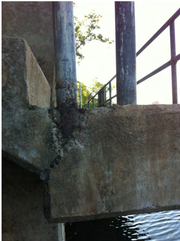
Figure 20. Catwalk handrail corrosion and concrete spall at Building B
