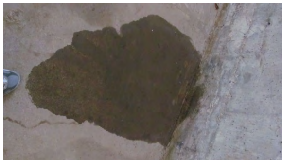
Figure 1. Leak in Basement Wall
