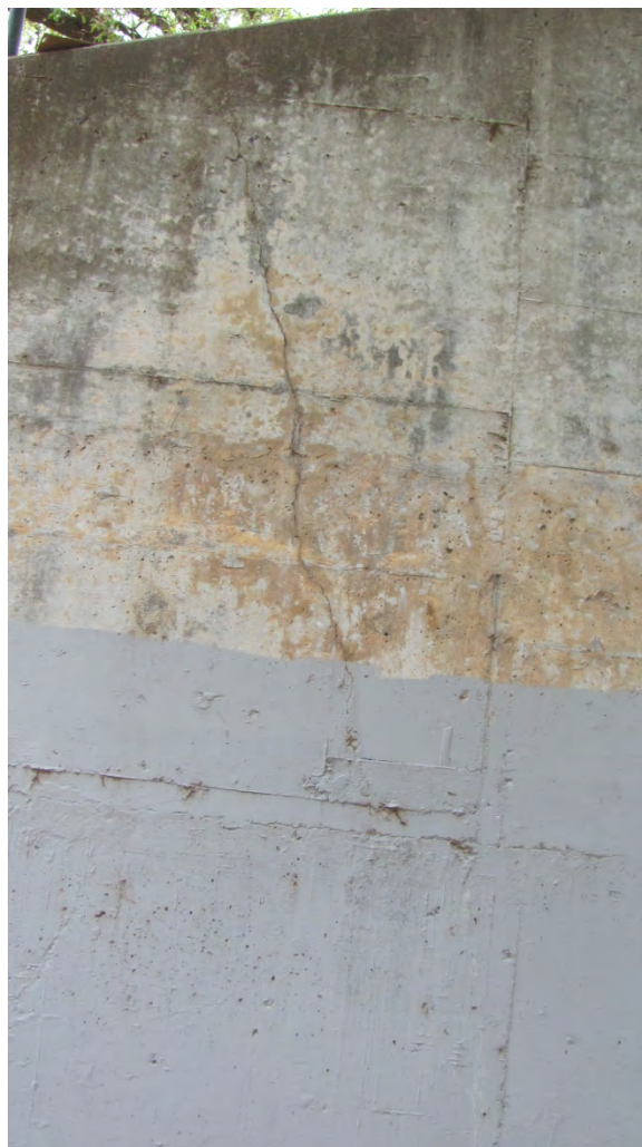
Figure 14. Diagonal crack in the retaining wall west of Building A
