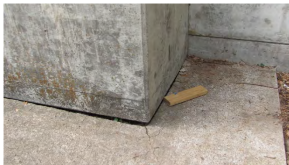
Figure 13. Sidewalk settling at the entrance to Building A
