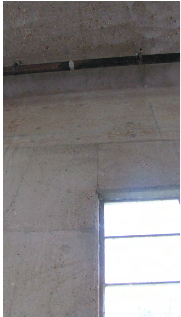
Figure 8. Horizontal construction joint at Building A
