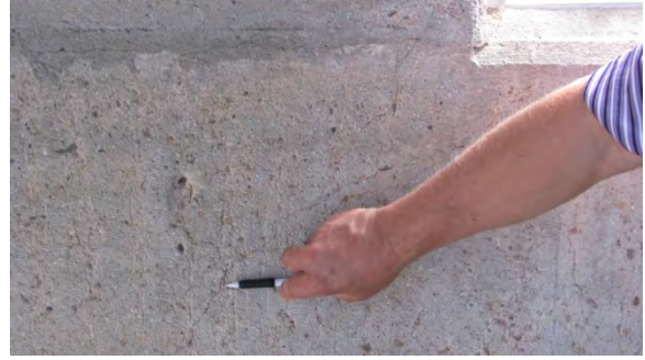
Figure 7. Diagonal crack at window in Building A
