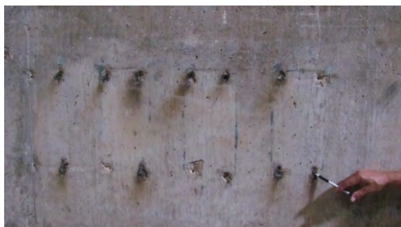
Figure 2. Embedded conduits in Basement wall
