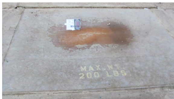
Figure 4. Metal cover over slab opening in Building A
