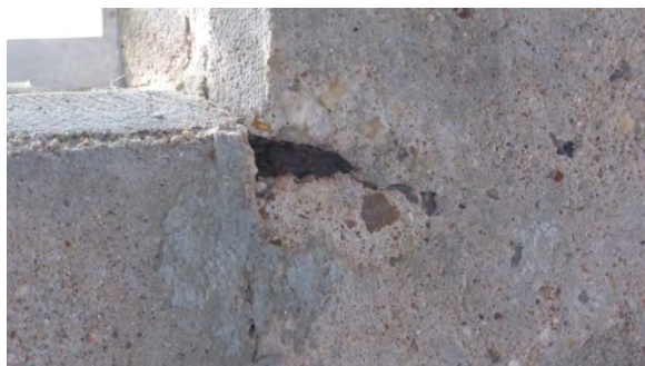
Figure 9. Spall with exposed reinforcement at Building A
