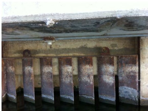
Figure 16. Corrosion of steel inlet gates at Building A
