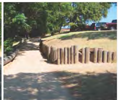
Deteriorating railroad tie retaining wall.
