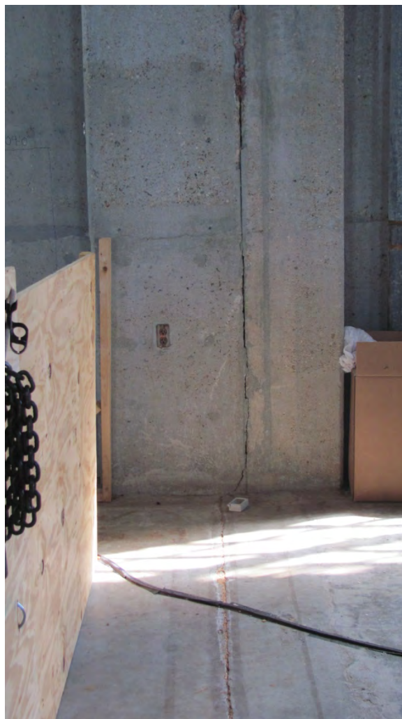
Figure 3. Building A.1/A.2 expansion joint
