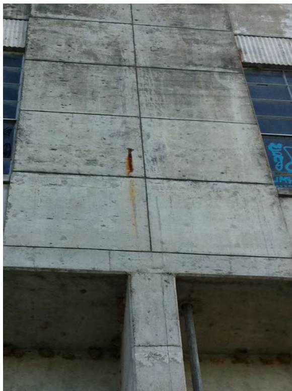
Figure 15. Exposed reinforcement in South wall of Building A
