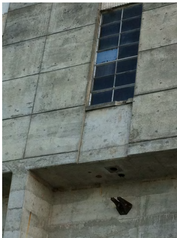
Figure 18. Spall at window sill at Building A
