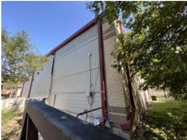
9. Partial west elevation.
