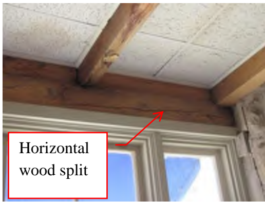
Figure 2. Sun Porch beams
