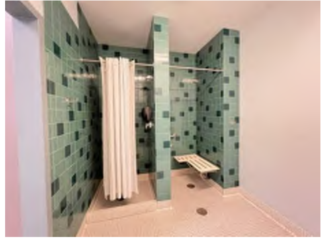
32. Main Building: Locker room shower finishes.
