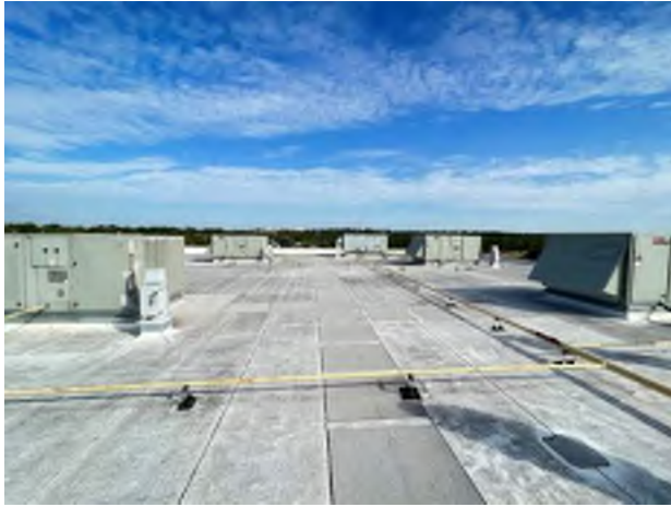
25. Multi-purpose Building: Overview of the roof.
