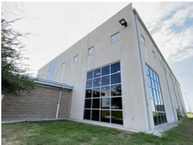
23. North and West elevations.
