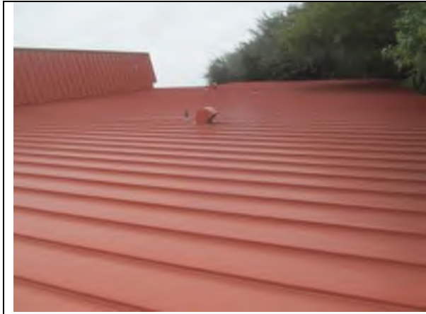
Overview of the roof.
