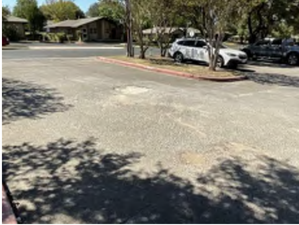
1. Pavement and Curbing
