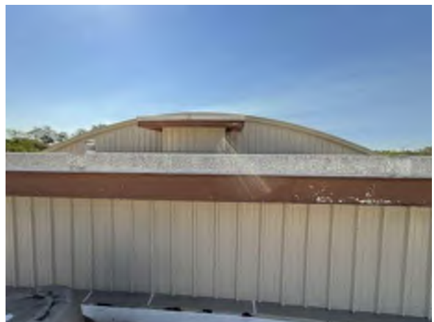
12. Standing Seam Metal Roof
