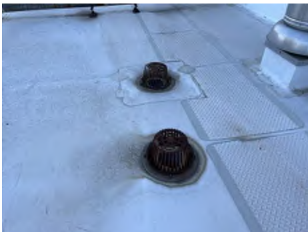
17. Roof and overflow drains
