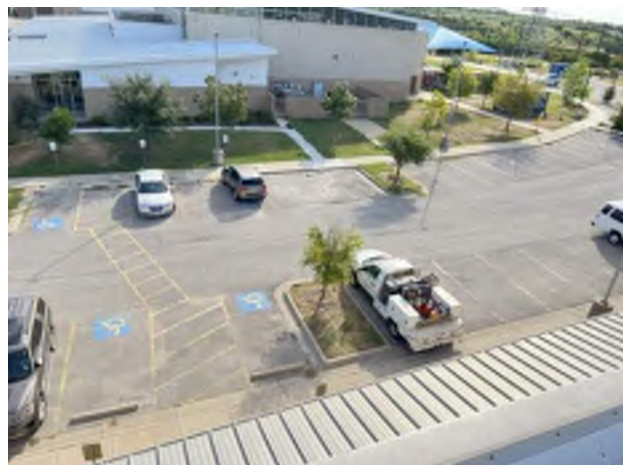
6. Asphalt paved parking lot
