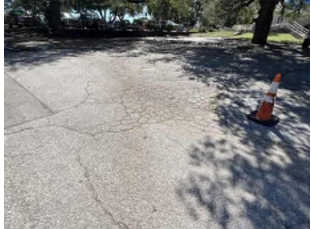
2. Asphalt parking lot
