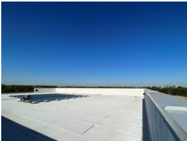
21. Upper roof overview.
