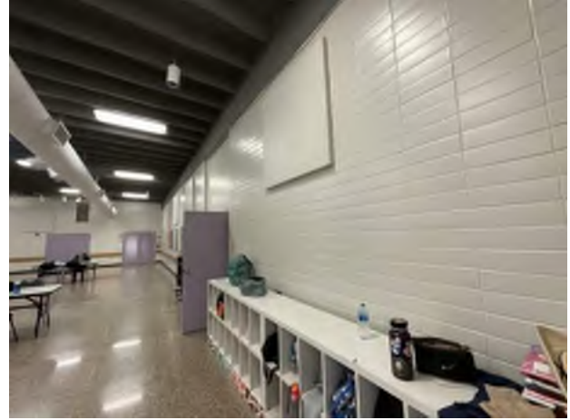
8. Subject: Multi Purpose Room
