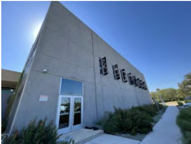
15. Partial west elevation.
