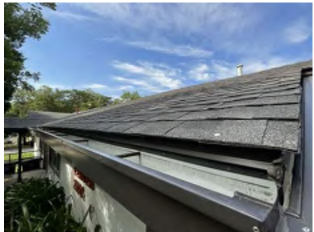
18. Roofing and Gutter
