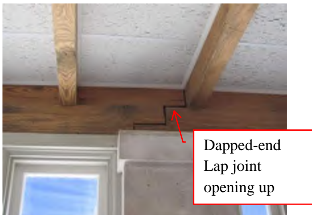
Figure 3. Sun Porch Beam/Column connection
