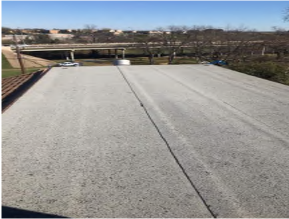
Small Modified roof area. No repairs needed.
