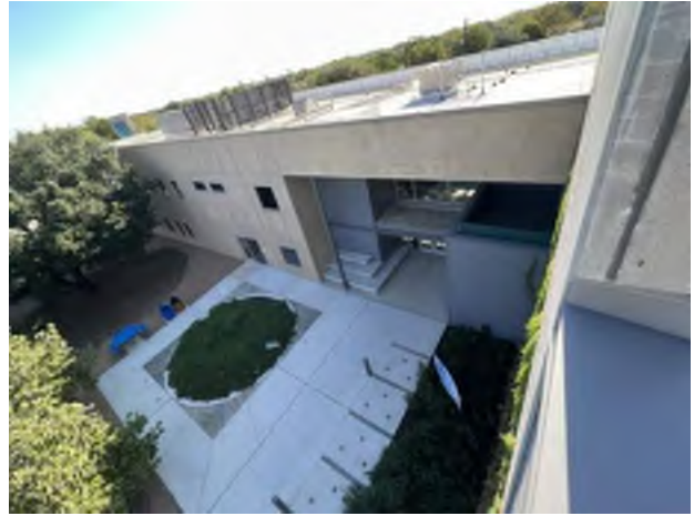
14. Partial west elevation.
