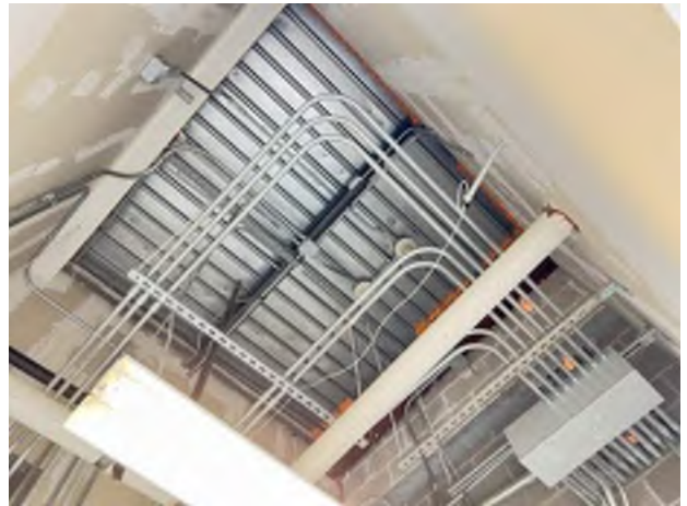
16. Metal Roof Deck
