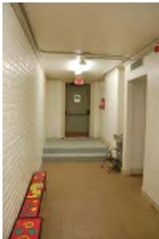
South interior lower level exit
