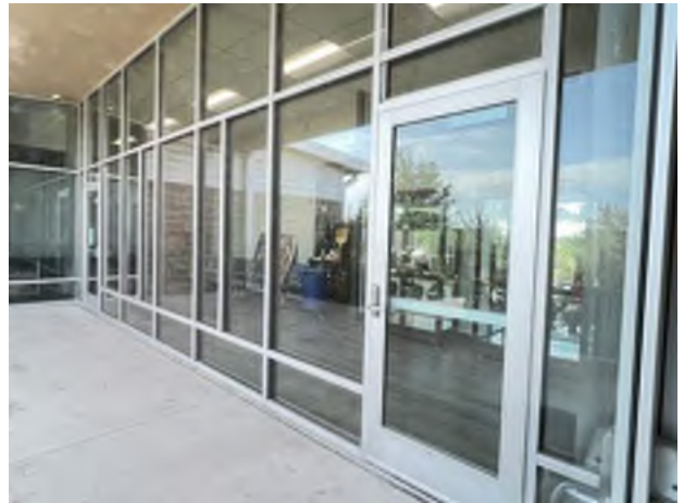
22. Main Building: Storefront glazing
