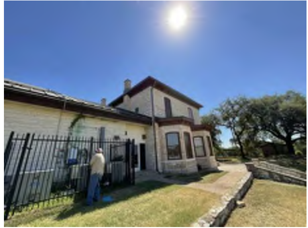
2. Retaining Wall and West Facade
