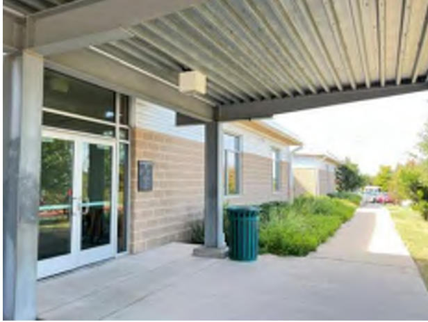
7. Main Building: Metal canopy and entry
