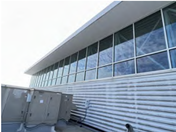
21. Main Building Clerestory
