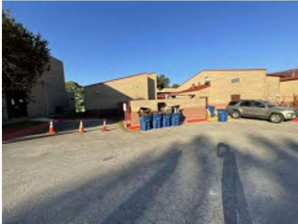
7. Southeast side of the property
