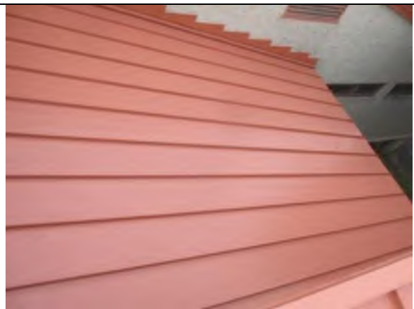
Overview of the roof.
