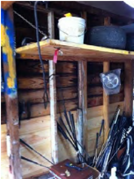
Figure 7. Cart Barn North Wall
