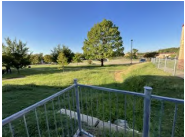
4. Storm Drain detention area
