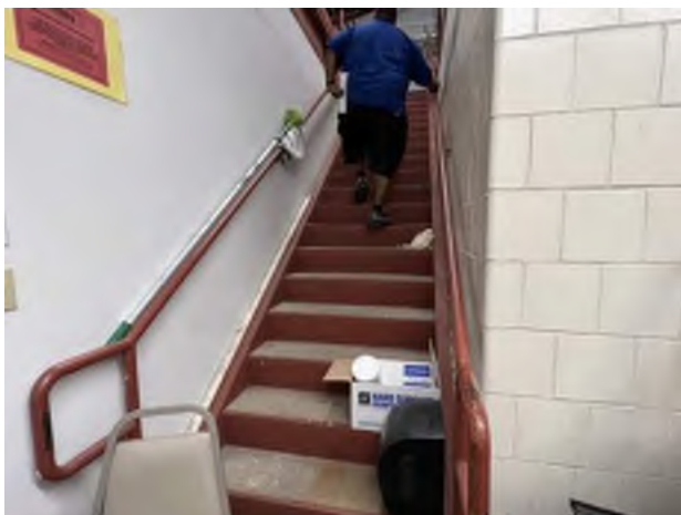
17. West mechanical attic stairs
