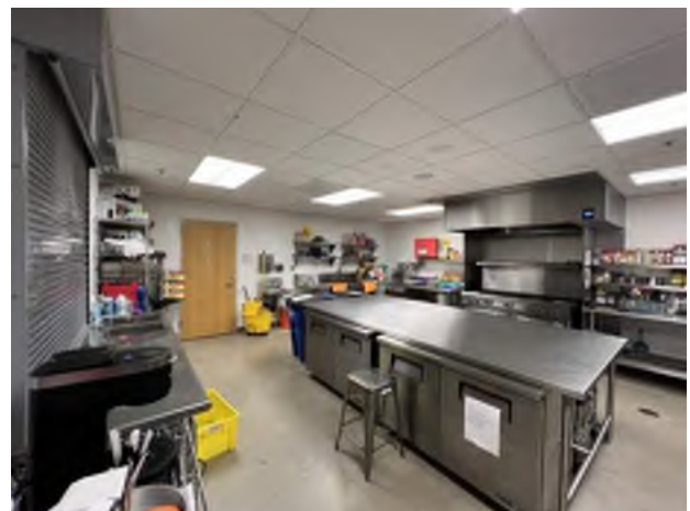
42. Kitchen interior finishes.
