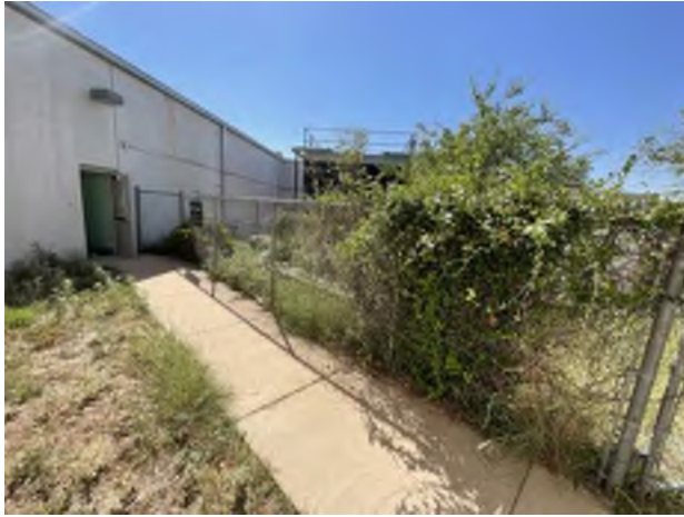
1. Typical Sidewalk at Rear Courtyard
