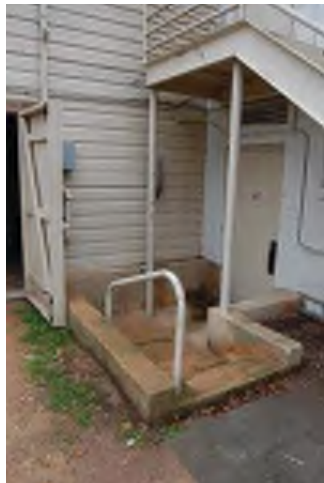
Northwest depressed entrance
