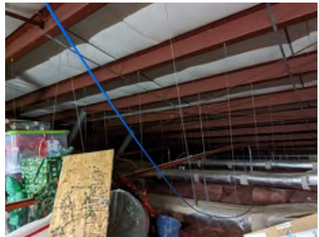
6. Steel Structure - Main Building
