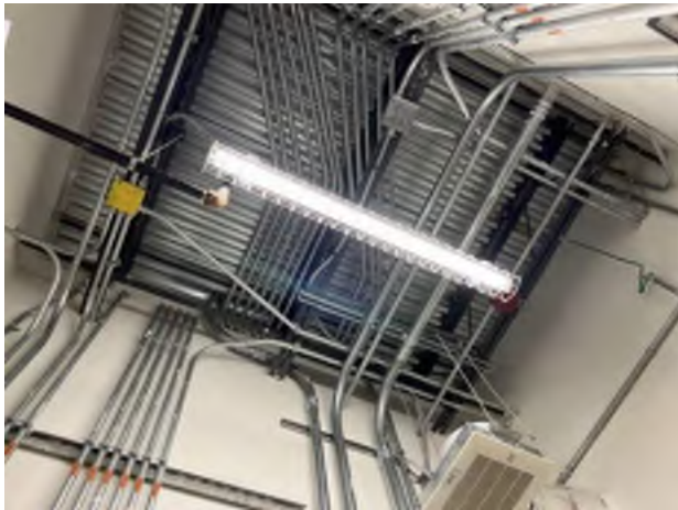
9. Metal deck structure
