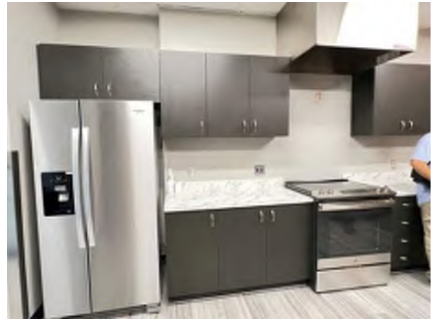
34. Main building kitchen finishes.
