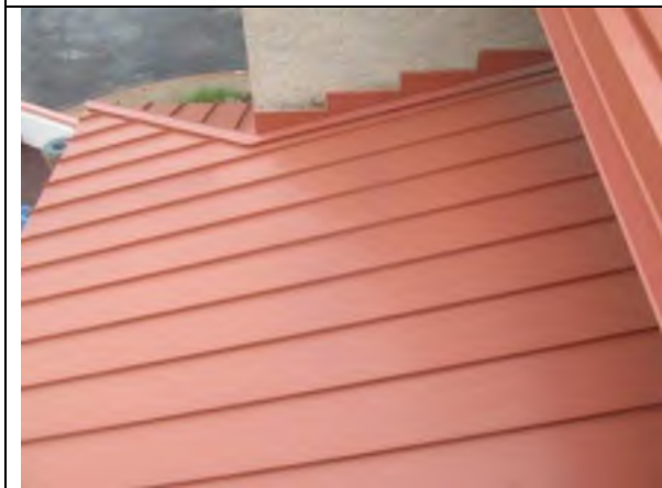
Overview of the roof.
