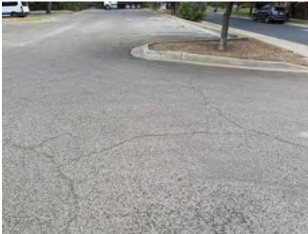
3. Asphalt Pavement with Concrete Curbing
