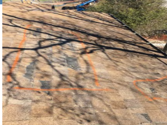
Shingle area marked.
