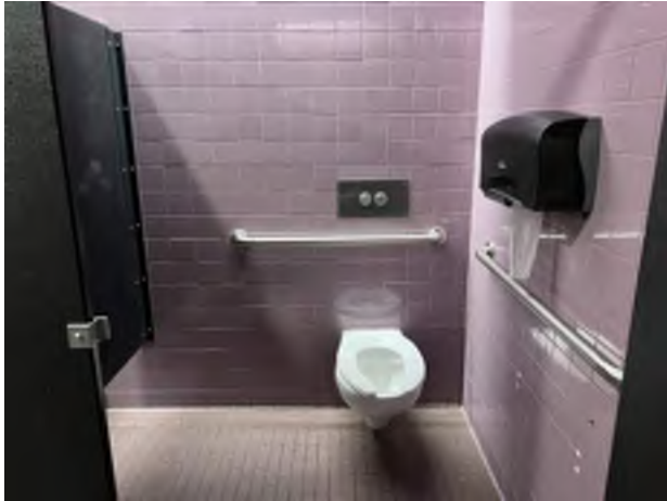
31. Typical ADA Accessible Toilet Stall
