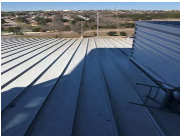
Area #2 No repairs needed. Next (7) pictures.
