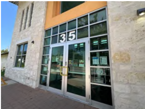
9. Storefront entry door.
