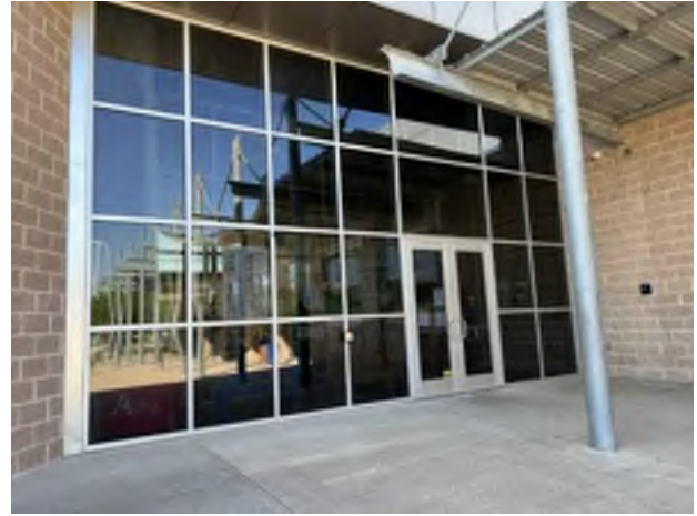
14. Main Entry Glazed Curtain Wall
