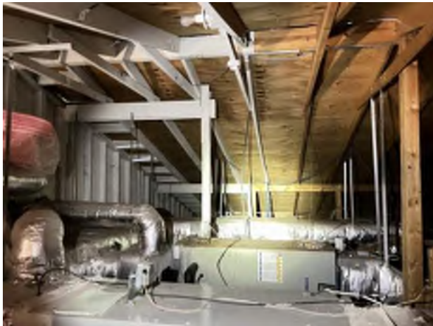
9. Wood-framed roof structure.
