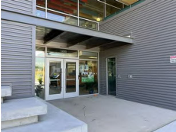
19. Main entrance doors.
