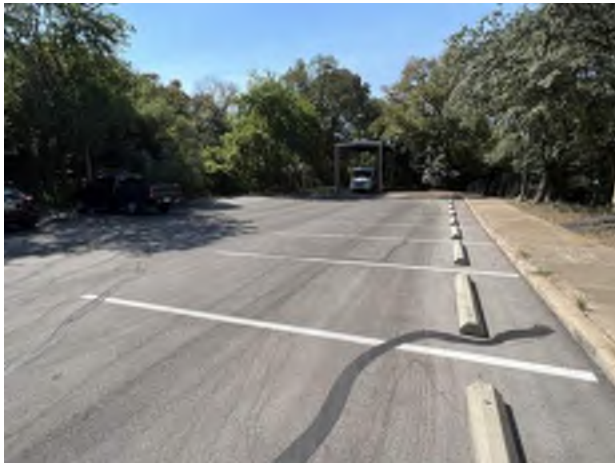
3. Asphalt parking lot
