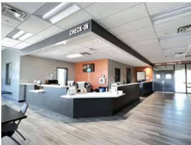
35. Main Building: Lobby interior finishes.
