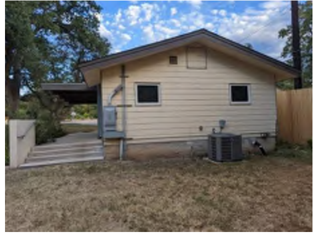
14. Annex Building - East Elevation
