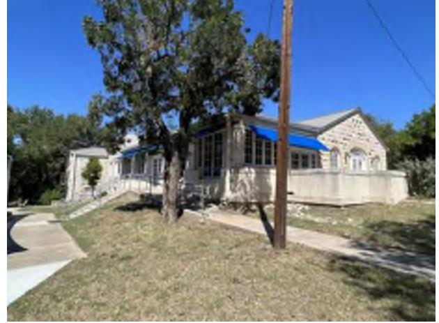
8. South and east elevations
