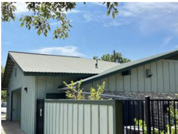
17. Pitched standing metal seam roof.
