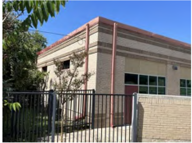
8. Southeast corner of the building.
