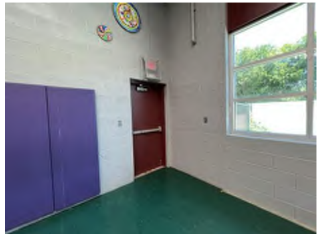
28. Illuminated exit sign at the gym exterior door.
