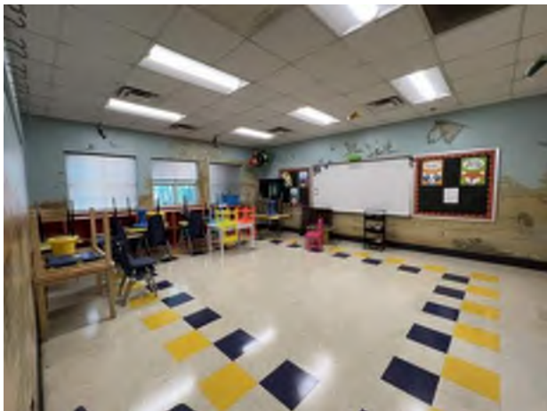
15. Representative classroom finishes.
