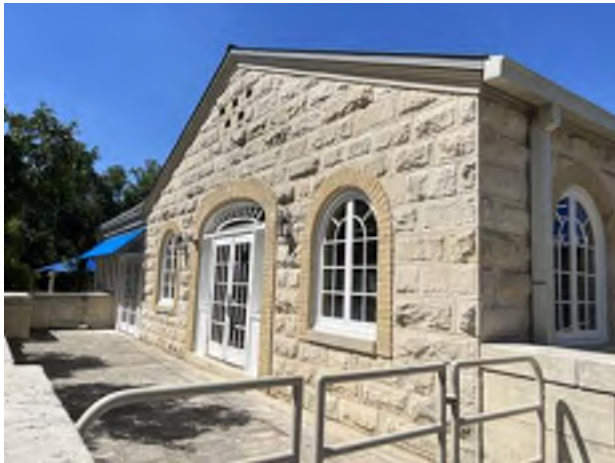
9. Exterior door and windows
