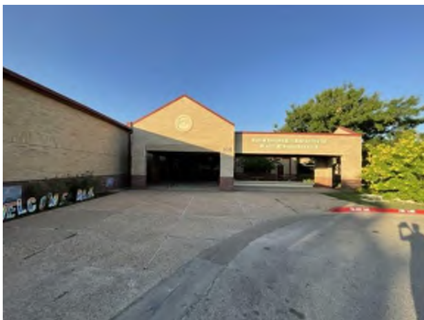
5. Front North Façade
