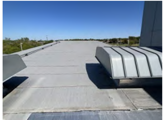
16. Lower Roof Field
