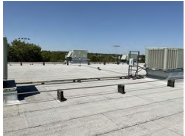
10. Built Up Roof
