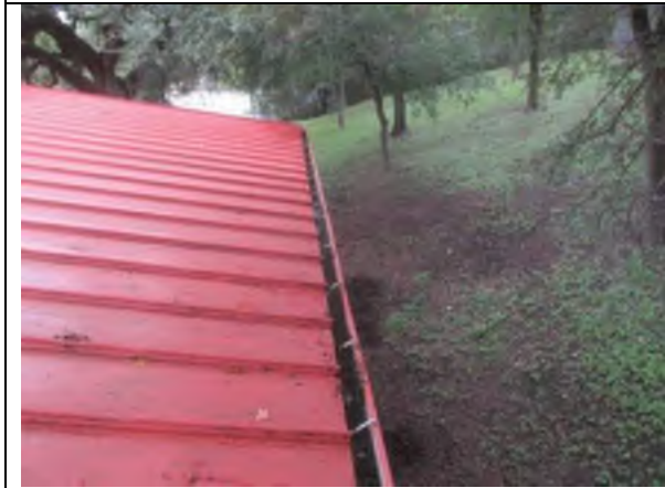
Overview of the roof.
