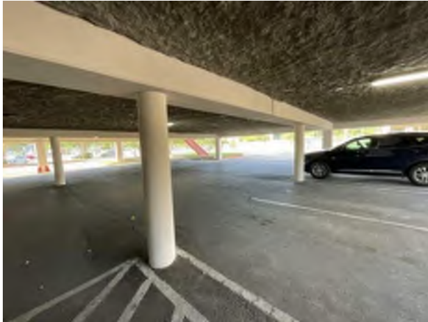
7. Parking Under the Building
