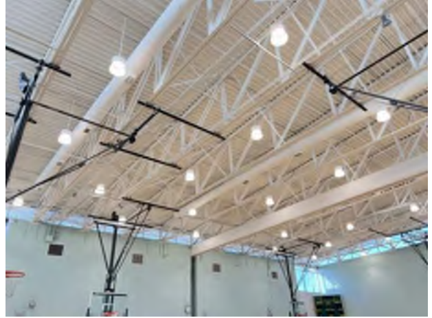
14. Main Building: Steel structure.
