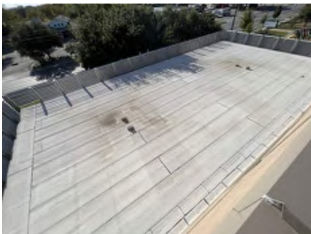
23. Lower roof overview.
