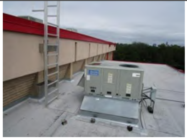
Overview of the roof.
