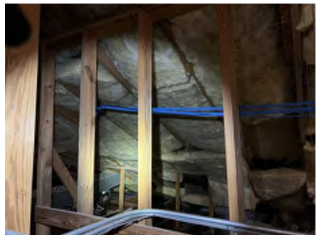
6. Wood-framed roof structure
