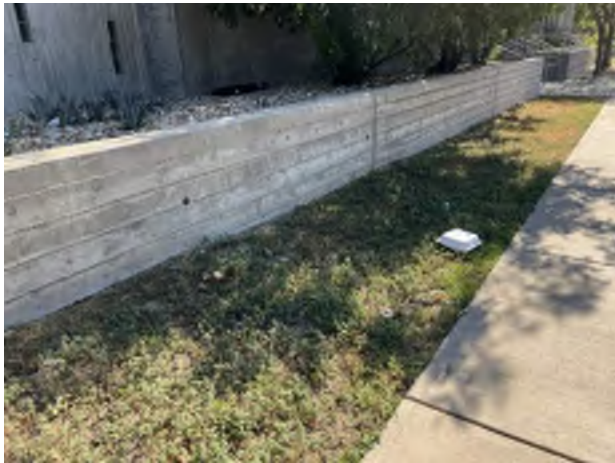
3. Concrete planter wall
