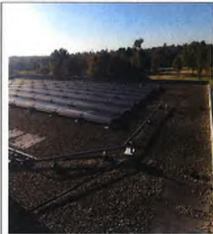
Gravel Built Up roof in Poor condition. Solar Panels installed in 2012.
