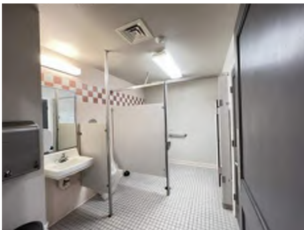
23. Restroom interior finishes.
