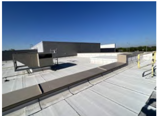
22. Middle roof overview.
