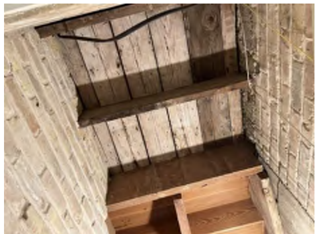
6. Wood deck framing
