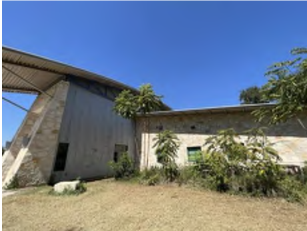
7. Partial east elevation
