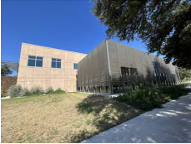
13. Partial east elevation.
