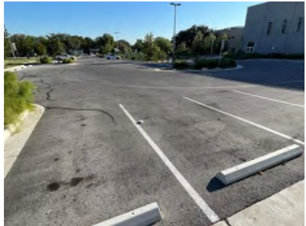
4. Asphalt parking lot.
