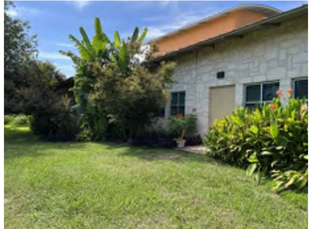
8. Partial south elevation.
