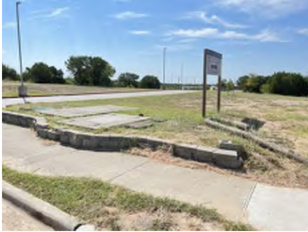
43. Water meters located off-site.
