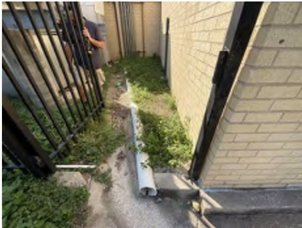
15. Roof Drain Leader
