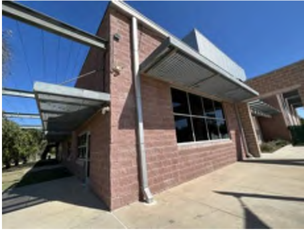
13. Exterior walls, eyebrows and downspout
