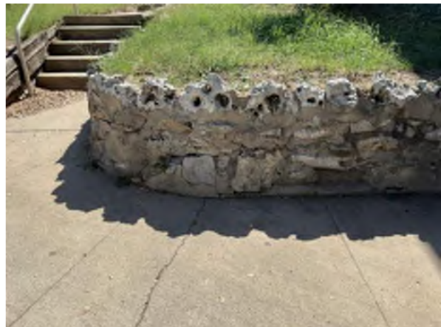
4. Stone retaining wall
