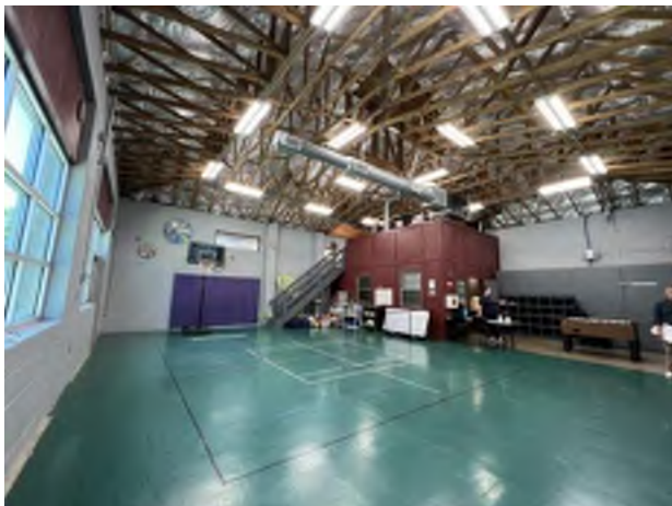
17. Gym interior finishes.
