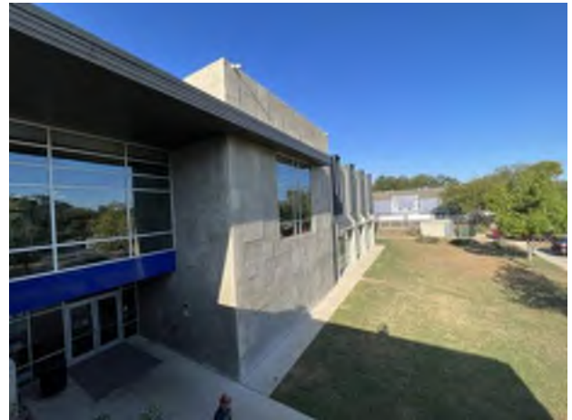
10. Partial north elevation
