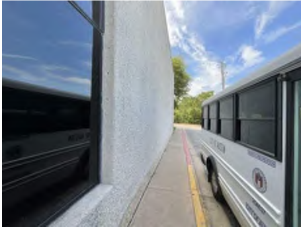
7. Exposed Aggregate Precast Concrete Wall Panel
