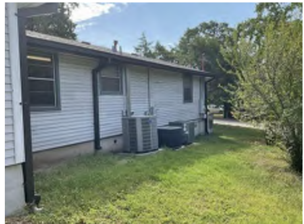
10. Façade with Condensing Units
