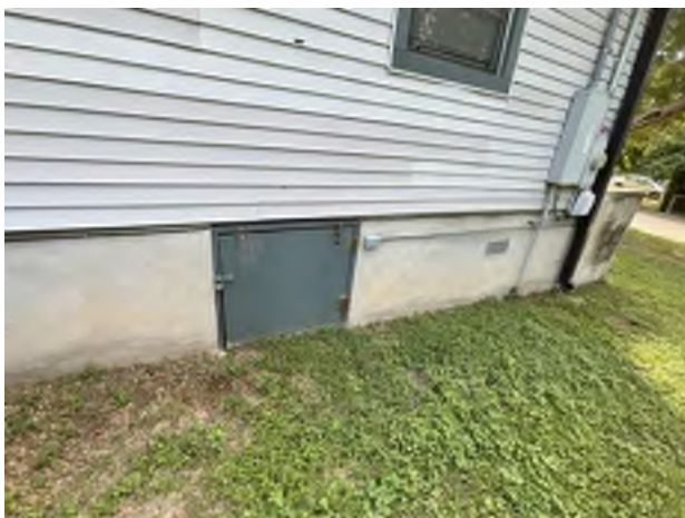
5. Concrete Stem Wall
