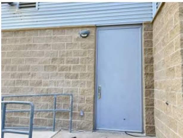
29. Multi-purpose Building: Service door.
