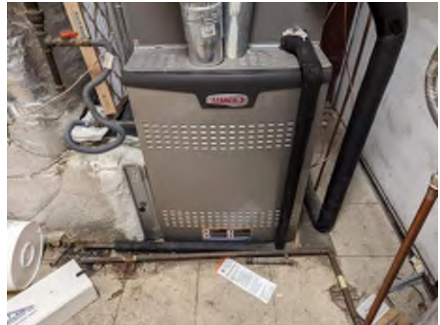
22. AHU at Main Building
