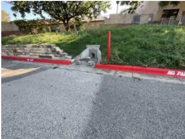
3. Retaining Wall and Culvert
