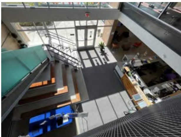
29. East lobby interior finishes.
