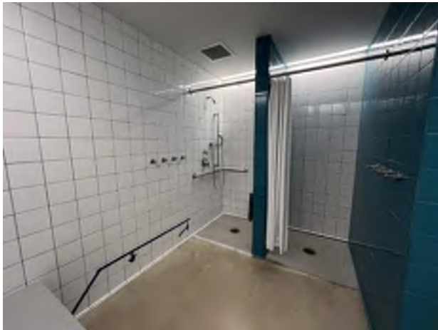
45. Women's shower interior finishes.
