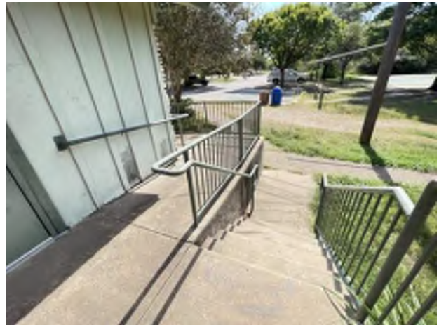
4. Exterior stairs and ramp
