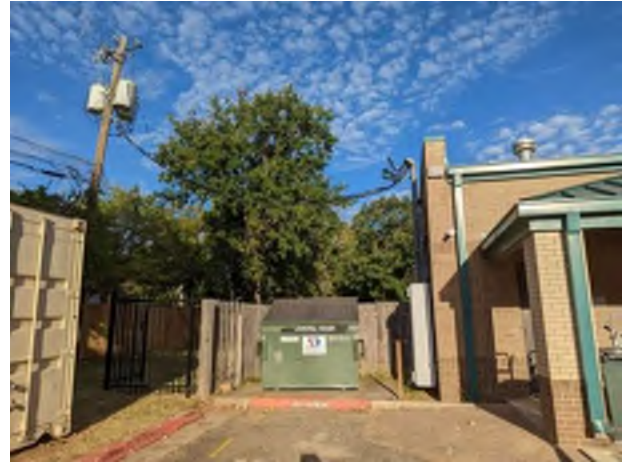
8. Trash Enclosure and Electrical Entrance
