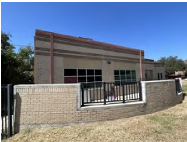
5. Brick site wall with painted metal fencing along the east side of the building
