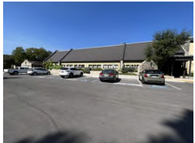
30. Accessible parking spaces
