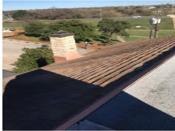
Shingle roof overview.
