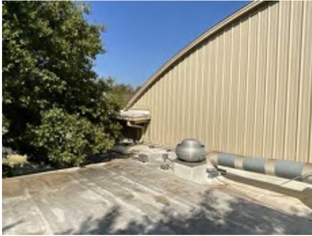
13. Metal Panel Walls
