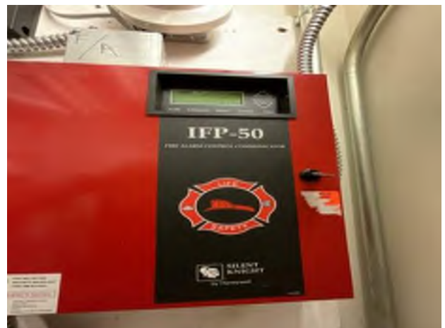
24. Annex: Fire Command
