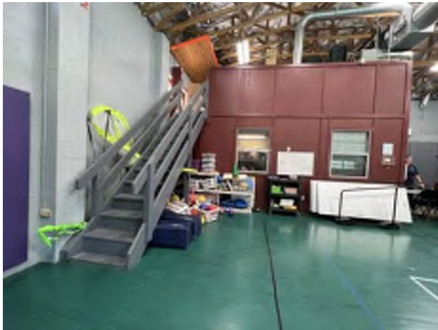
21. Interior stairs at the storage and mechanical loft
