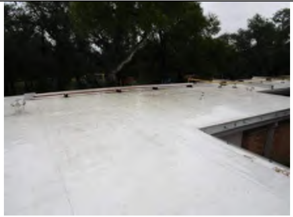
Overview of the roof.
