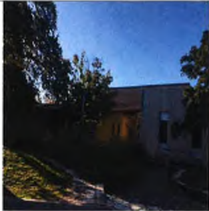
2913 Nrothland Dr. Modified roof installed in 2011. Good Condition.
