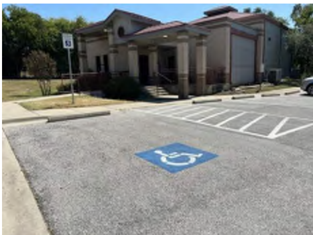
29. Accessible parking space with access aisle at the parking lot
