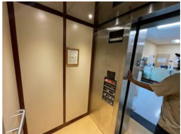
24. Interior Cab Finishes
