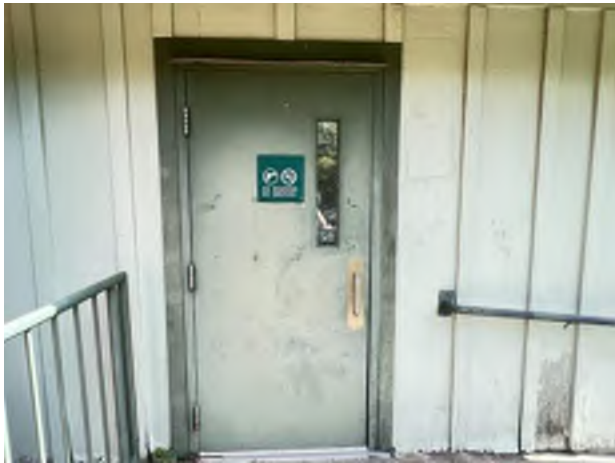
15. Painted hollow metal exterior door.
