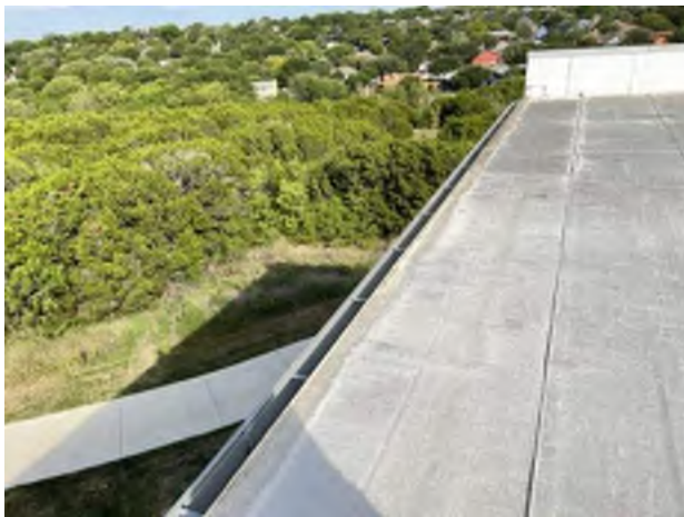
27. Multi-purpose Building: Gutter
