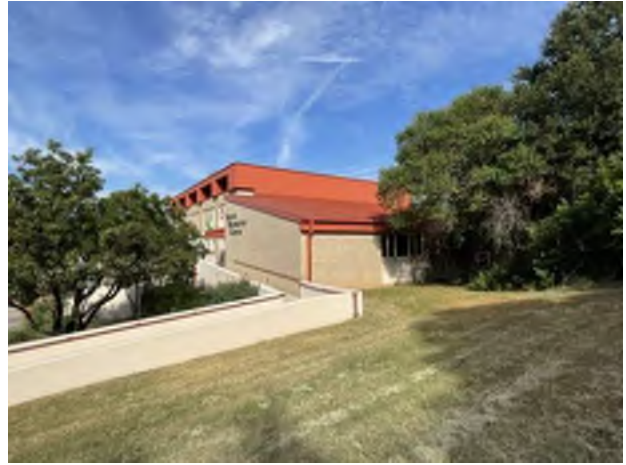
2. East Façade Yard
