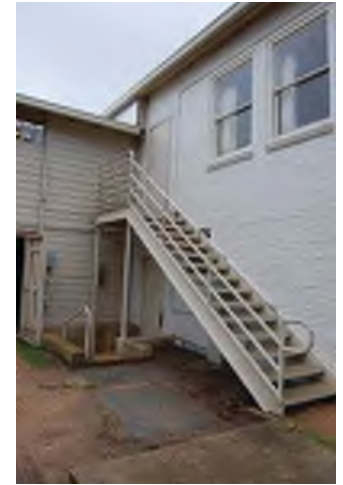
Existing north stair
