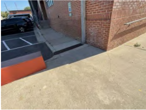
1. Parking ,Curbing, and Sidewalks
