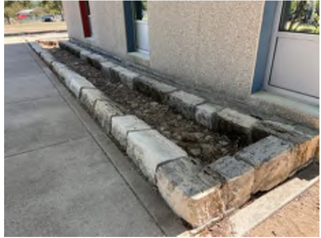
2. Decorative drainage feature
