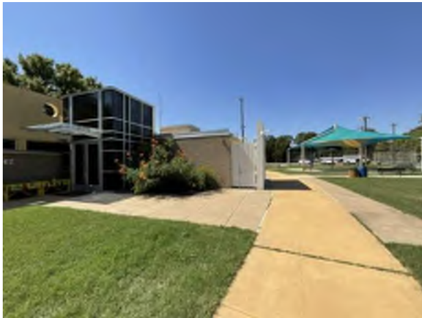
15. Main Entrance and MEP Yard
