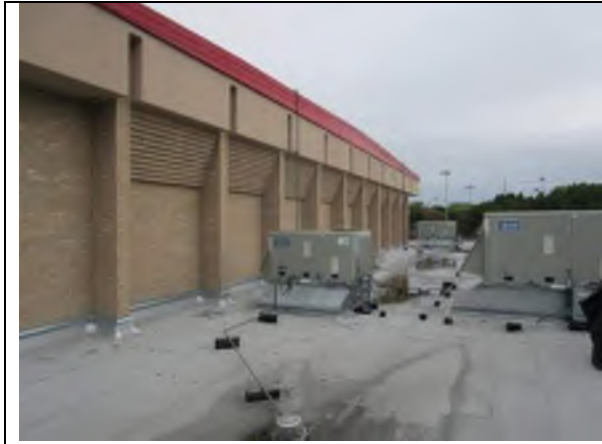
Overview of the roof.
