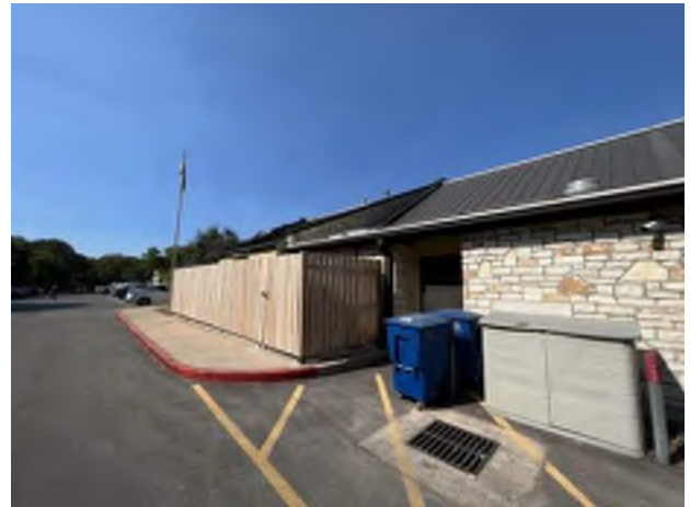
4. Catch basin and wood fencing
