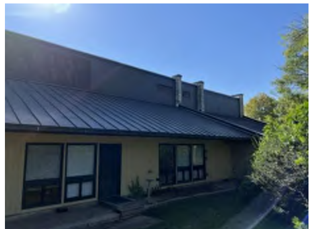
12. Standing metal seam roof
