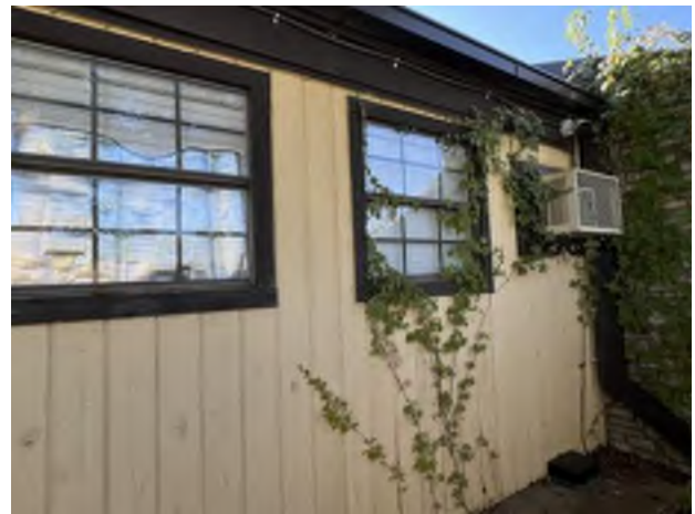
10. Wood siding and wood framed windows
