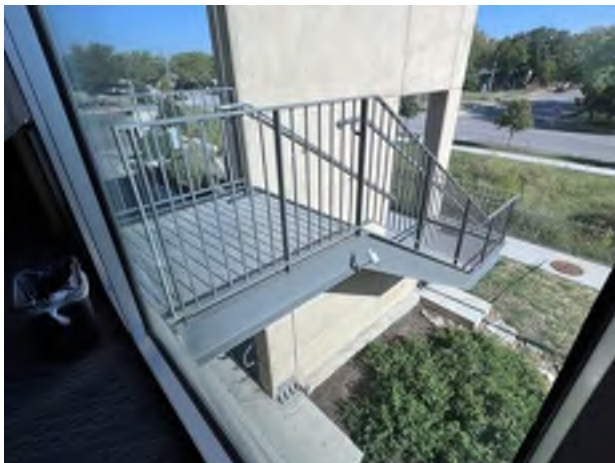
17. Exterior painted metal stairs.
