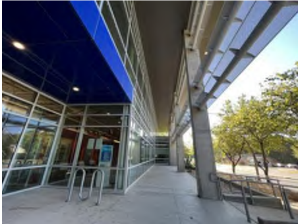
13. Storefront window system at south elevation
