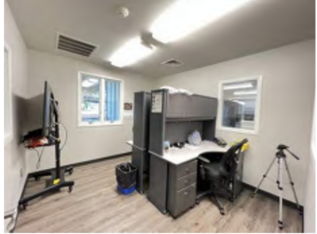
20. Office interior finishes.
