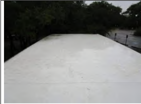
Overview of the roof.
