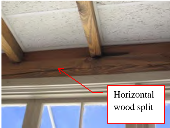
Figure 1. Sun Porch beams
