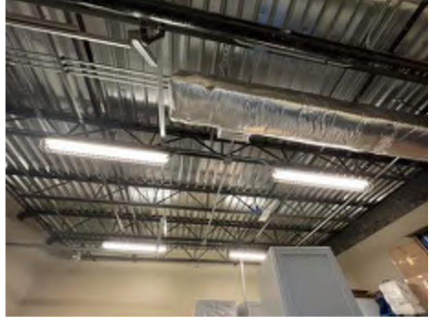
8. Metal roof structure
