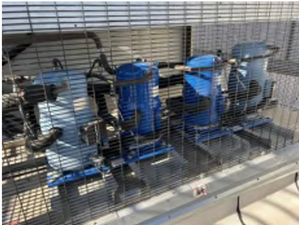
51. Replaced condenser at RTU-2.
