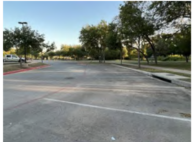
4. Asphalt parking lot
