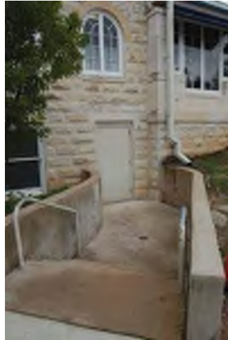
Existing south lower level exterior exit
