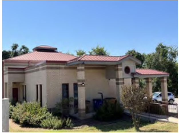
14. Pitched standing metal seam roof.
