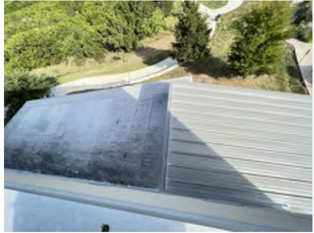
26. Multi-purpose Building: Roofs
