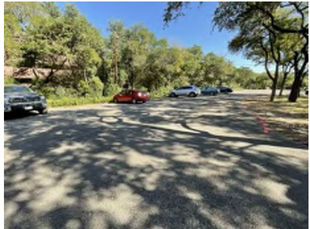
4. Subject: Pavement Area
