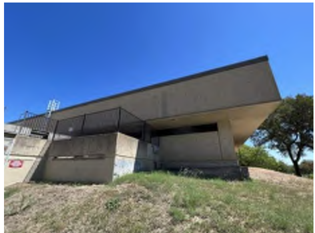
12. Partial west elevation
