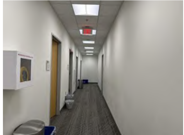
32. Corridor interior finishes.
