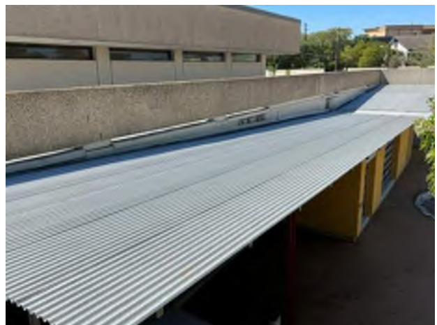
18. Metal roof at the Entry
