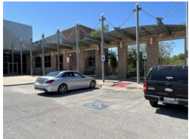
46. Accessible parking stalls and accessible path
