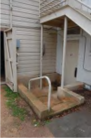
Existing north lower level exit
