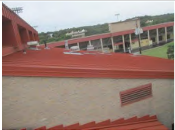
Overview of the roof.
