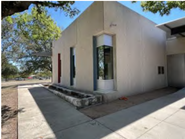
9. Partial north elevation
