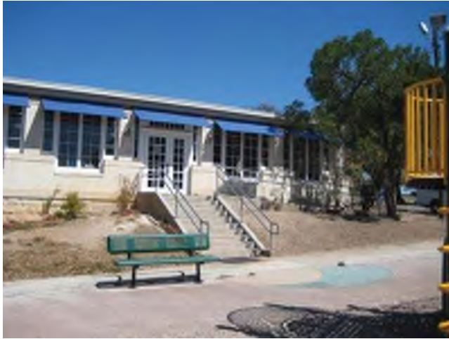
South entrance stair
