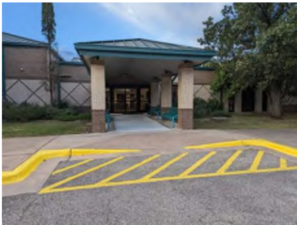
9. Front Entrance Canopy
