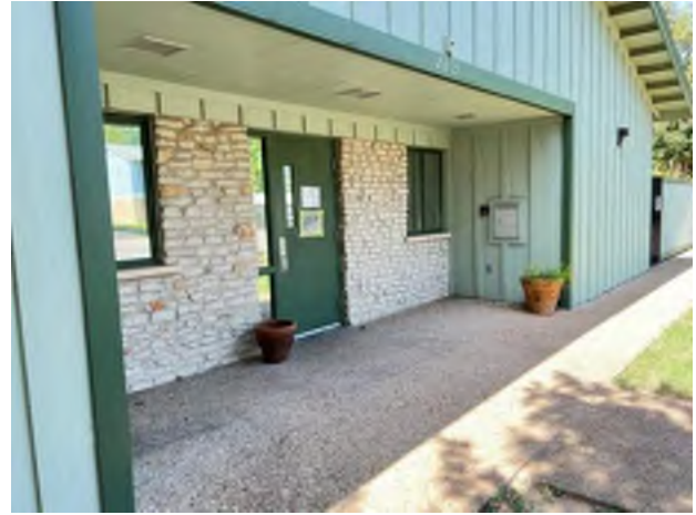
14. Main Building Entrance.
