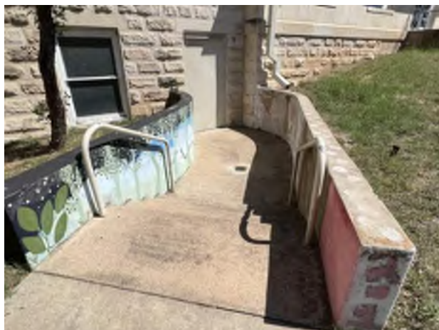
5. Low retaining walls
