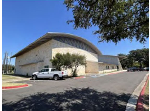
8. West and south elevations
