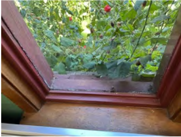
13. Single-pane exterior windows with painted wood frames.
