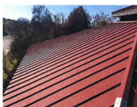
Next (5) pictures are of overview of Metal roof area.
