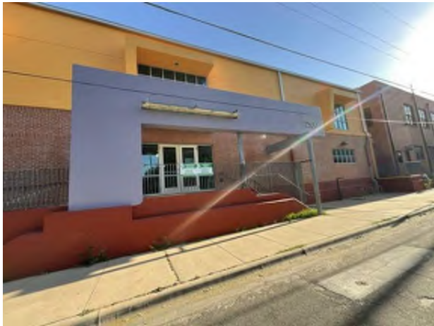
3. Front Entrance along 3rd Street
