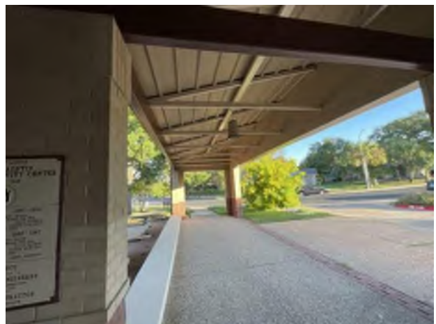
6. Drop Off Canopy
