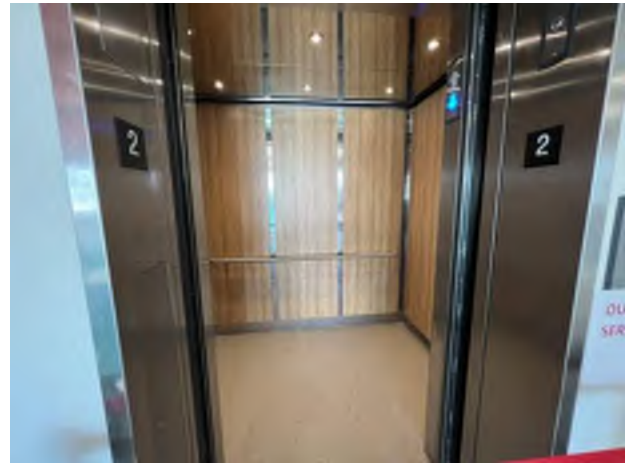
64. Elevator cab finishes.
