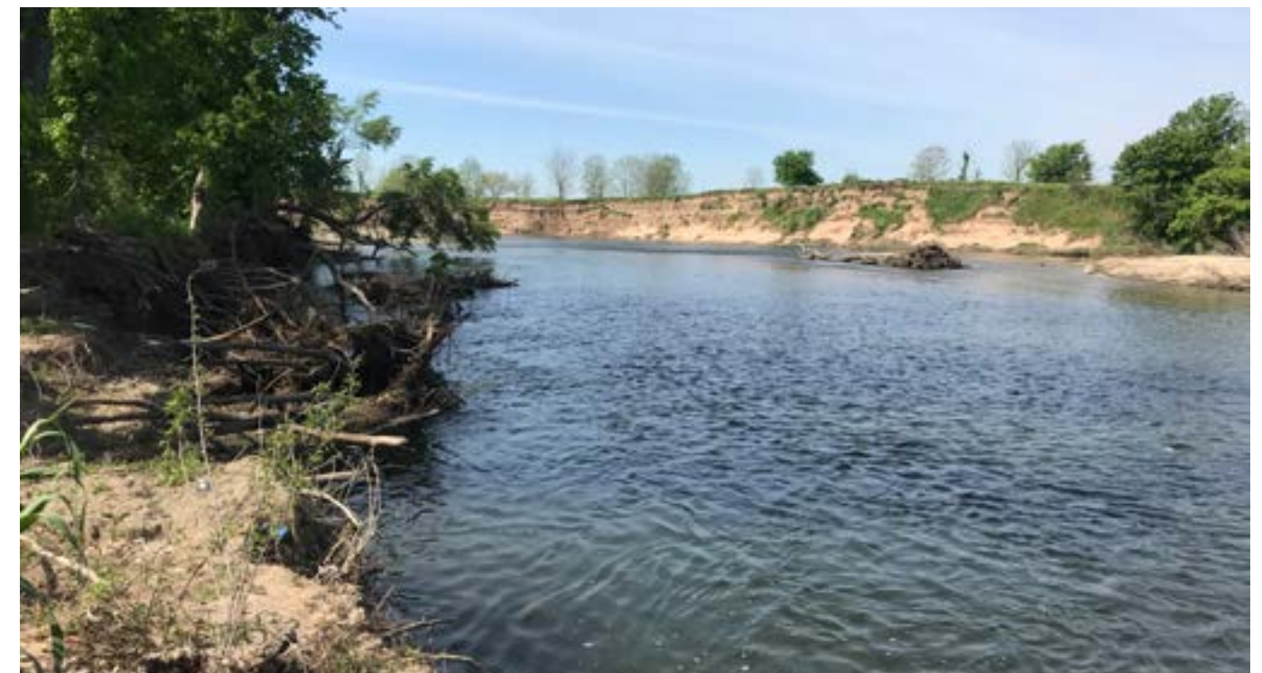
The dynamic movement of the Colorado River actively shapes the southern edge of Treviño Park (Image credit: Siglo Group)
