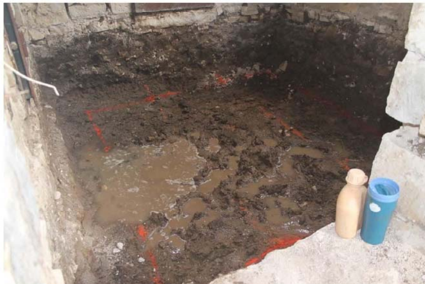
Figure 12: Room in northeast corner of the chapel inundated with water 1/13/17.
