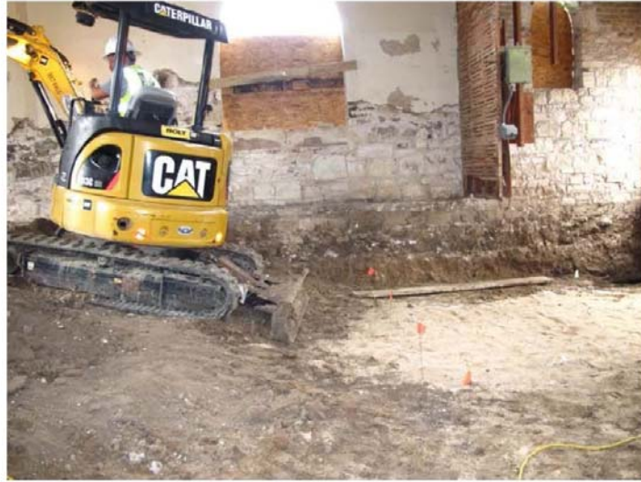
Figure 2: Mechanical operations within the chapel, note protective sand in plastic lined XU1-7.
