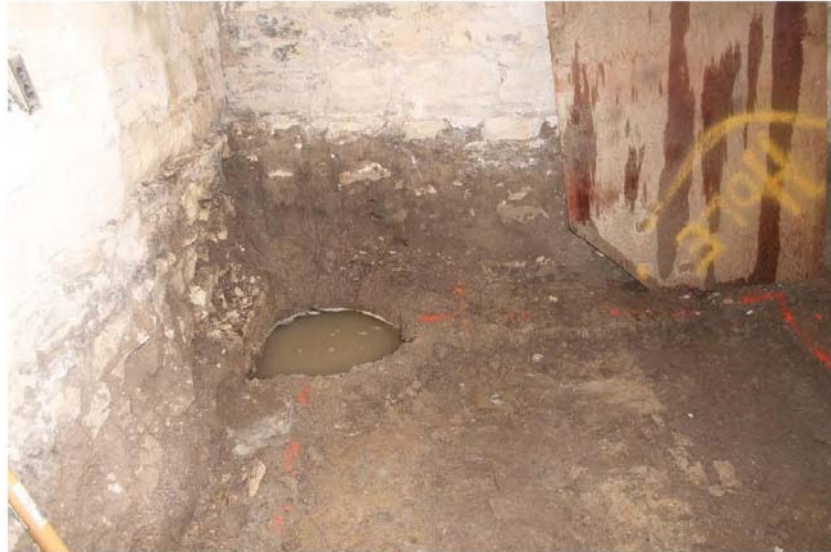
Figure 11: Pier hole in northeast corner of tower filled with water 1/13/17.
