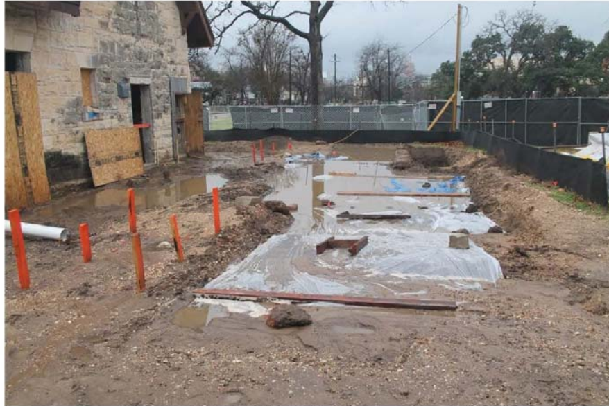
Figure 9: Blocks A-D filled with water after rain on 1/13/17.
