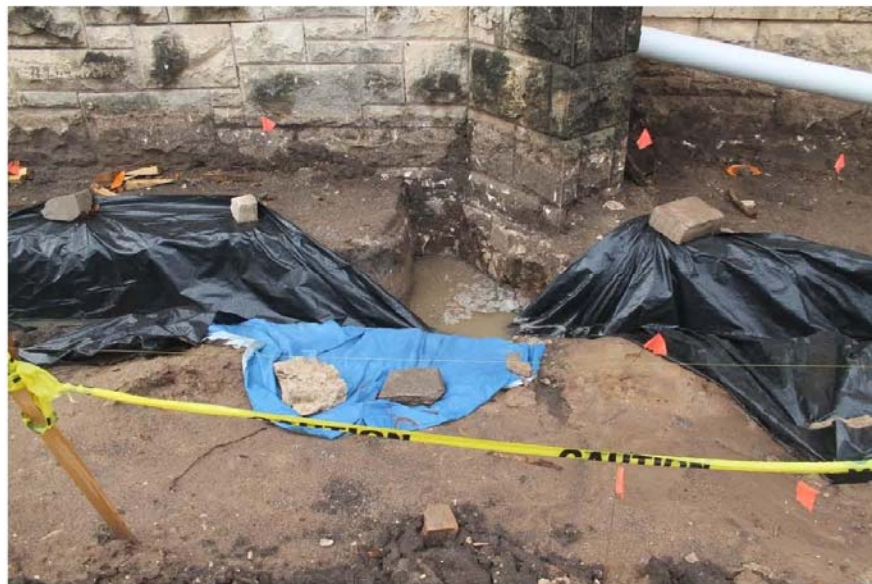
Figure 10: Outside Trench 1 filled with water on 1/13/17.
