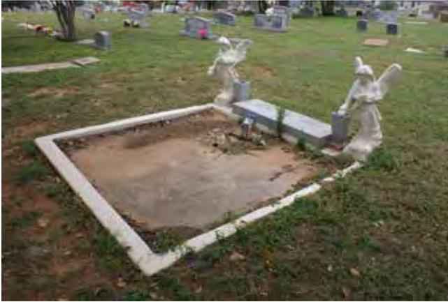
Figure 400. Concrete curbing enclosing a plot (McDoux Preservation)
