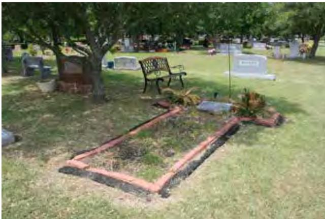
Figure 522. Plot curb made of brick paving units (John Milner Associates)
