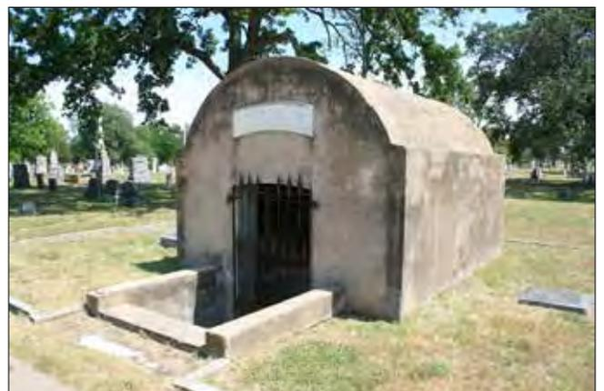
Figure 195. The concrete-stucco-clad, brick masonry Kreisle mausoleum in Section 1 (John Milner Associates)
