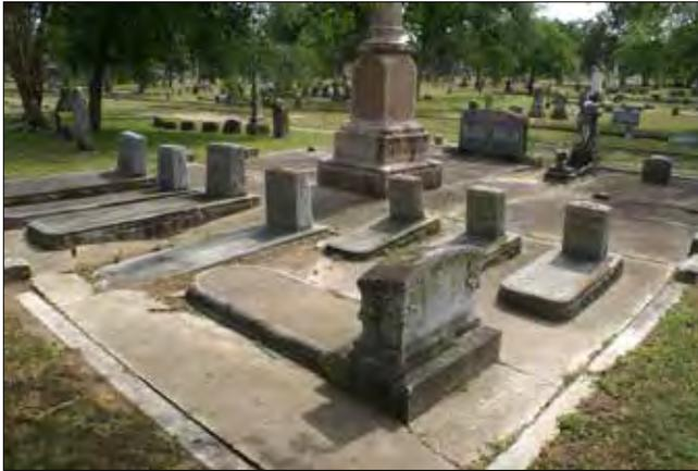
Figure 130. Concrete slab poured over crypts and plot (McDoux Preservation)
