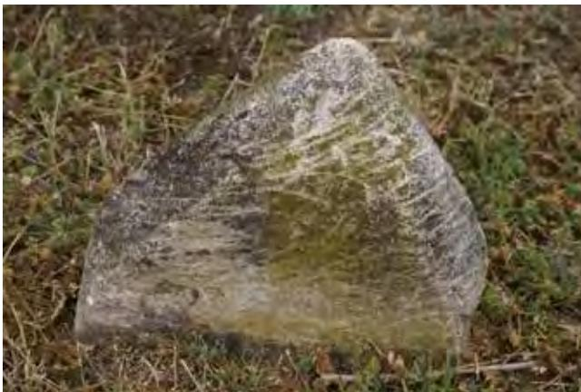
Figure 385. Marker damaged by trimmers (McDoux Preservation)
