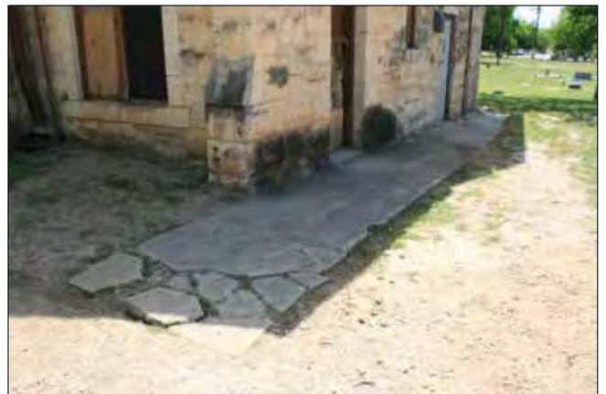
Figure 69. A concrete sidewalk leading to the chapel restroom is similarly in poor condition. (John Milner Associates)
