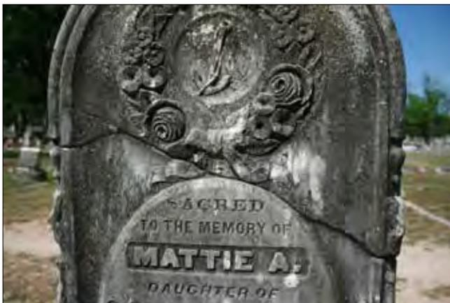
Figure 126. Previously repaired tablet marker (JMA\_050114\_0366)
