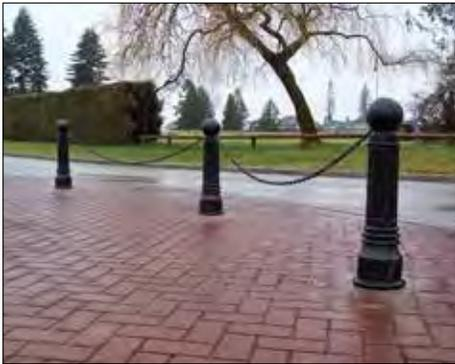
Figure 221. Steel bollards with chain
