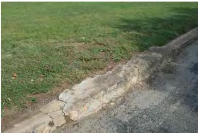
*Figure 449. Poor repair of the rock curb lining the entrance drive (John Milner Associates)*
