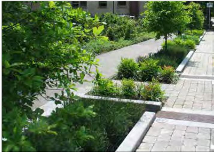
Figure 217. Adaptive re-use of the drainage channel as a bioswale planter is an option, as shown in this example. (EPA.gov)
