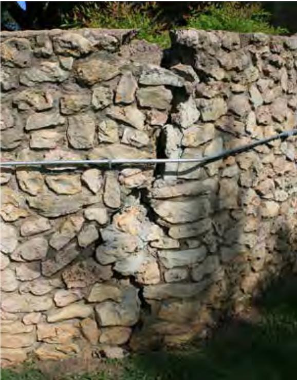
*Figure 536. Severely cracked portion of the wall, with attempted repair visible below the steel conduit (John Milner Associates)*
