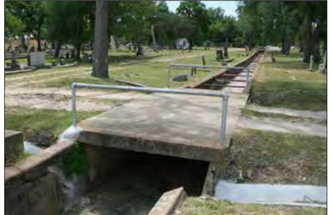
*Figure 61. A concrete vehicular bridge crossing the drainage channel (John Milner Associates)*
