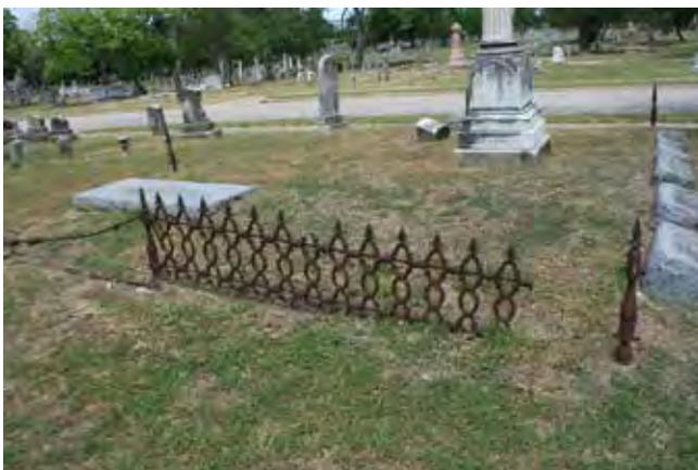
Figure 170. Cast iron fencing, with many missing sections (John Milner Associates)
