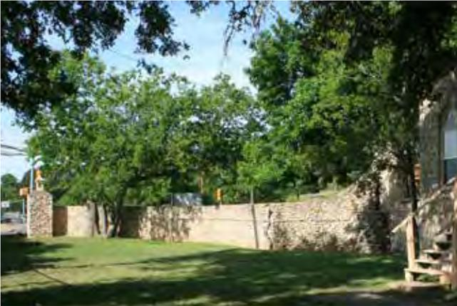
*Figure 535. Limestone retaining wall (John Milner Associates)*
