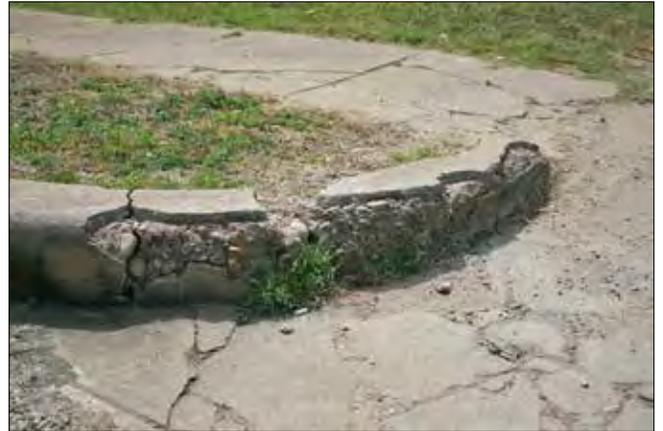
Figure 65. Turning vehicles have caused severe damage to this curb. (John Milner Associates)
