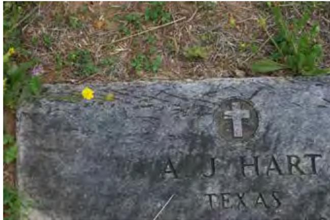
Figure 326. Mower damage to a flush marker (McDoux Preservation)
