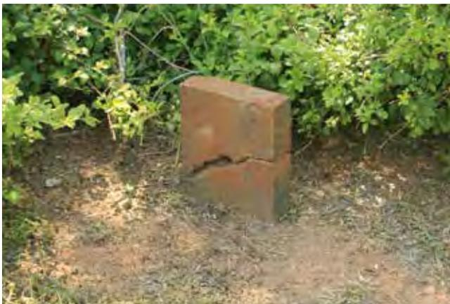
Figure 329. Cracked marker (John Milner Associates)
