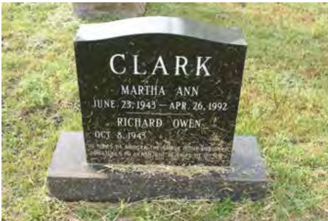
Figure 274. Grass clippings piled at the base of a marker and stuck to the surface (McDoux Preservation)
