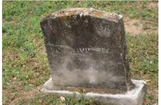
Figure 384. Both the base and face of this marker are damaged by trimmers (McDoux Preservation)
