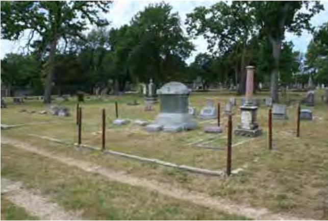
Figure 166. The cast iron fencing has been removed, leaving only the support posts. (John Milner Associates)
