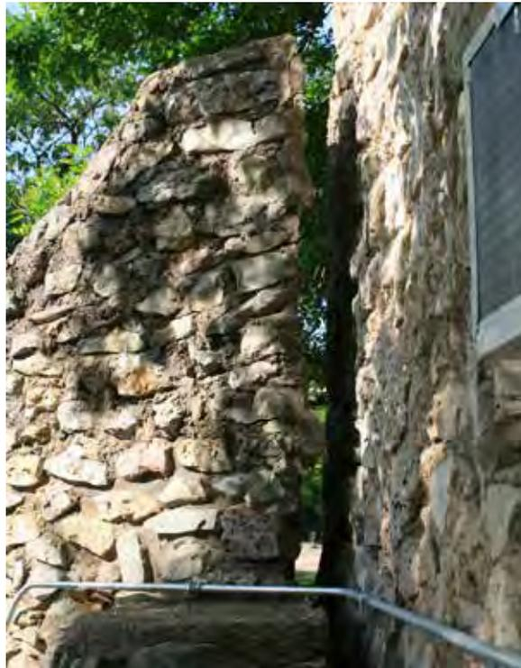
*Figure 537. The wall has completely separated from the adjacent building. (John Milner Associates)*
