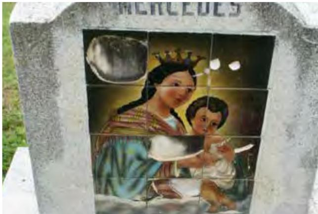
Figure 508. Damage to tile from rocks thrown by mowers (McDoux Preservation, AM-DSC08676)
