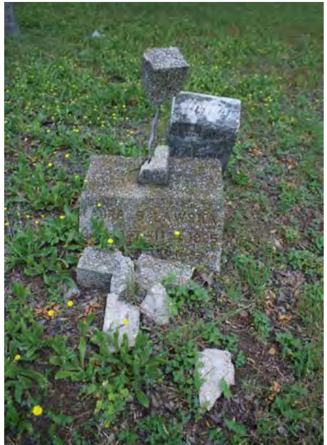
Figure 322. Broken concrete cross (McDoux Preservation)
