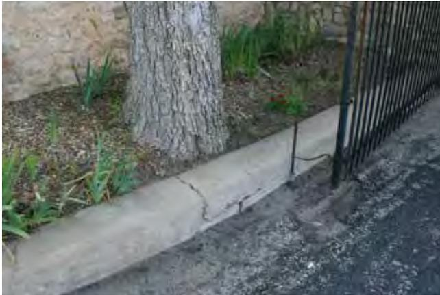
Figure 451. A cracked portion of concrete curb, just inside the entrance gate; the cracking is likely due to pressure from the adjacent pecan tree, which probably is a volunteer, rather than having been planted there. (John Milner Associates)
