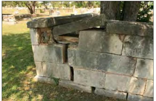
*Figure 165. The wall is severely cracked, and has missing and displaced stones. (John Milner Associates)*
