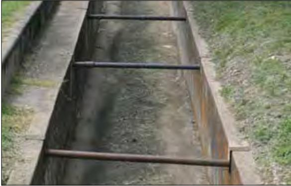
Figure 216. The dark, weathered surface of these steel spacers is ideal for minimizing glare, reflection, and visibility in the landscape. (John Milner Associates, 2014)
