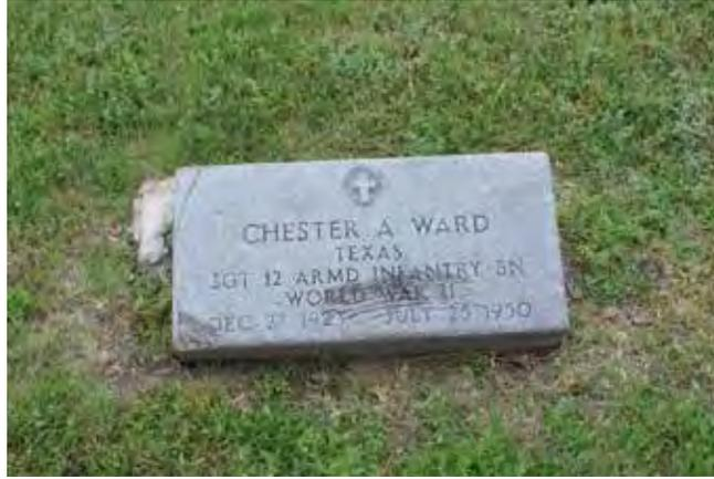
Figure 507. Trimmer damage to a VA marker (McDoux Preservation, AM-DSC08707)
