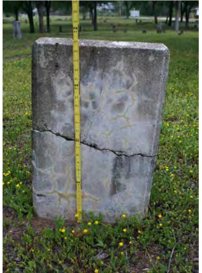
Figure 328. Cracked marker with visible repairs (McDoux Preservation)
