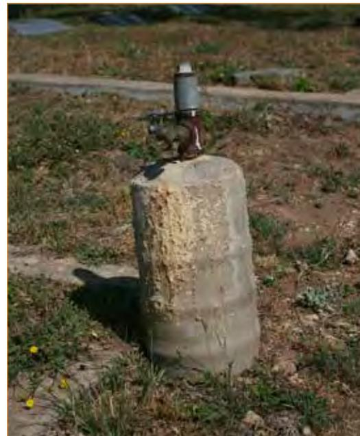
Figure 188. Iron pipe riser with mineral deposits (John Milner Associates)
