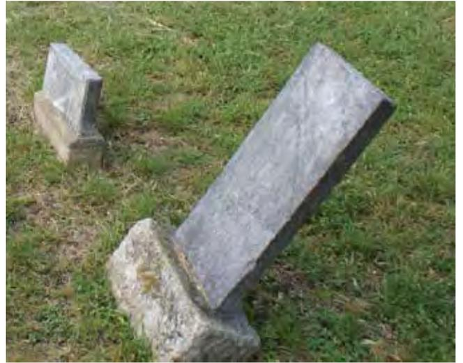
*Figure 267. Severely tilted marker (McDoux Preservation)*
