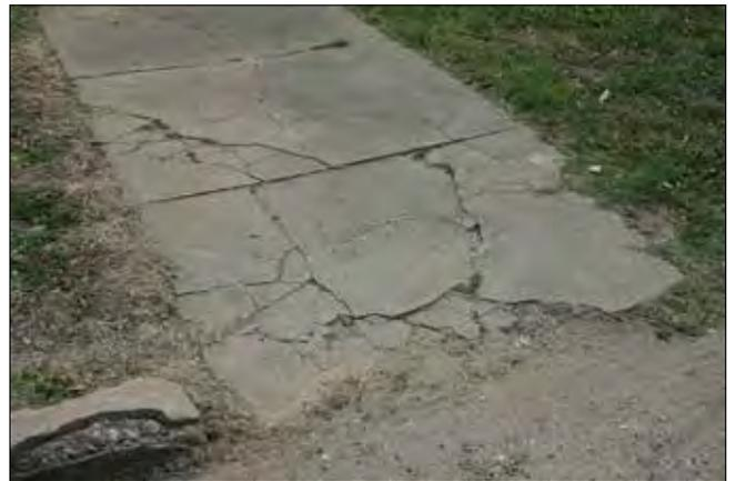
Figure 67. Many portions of the sidewalk lining Main Avenue are in poor condition. (John Milner Associates)
