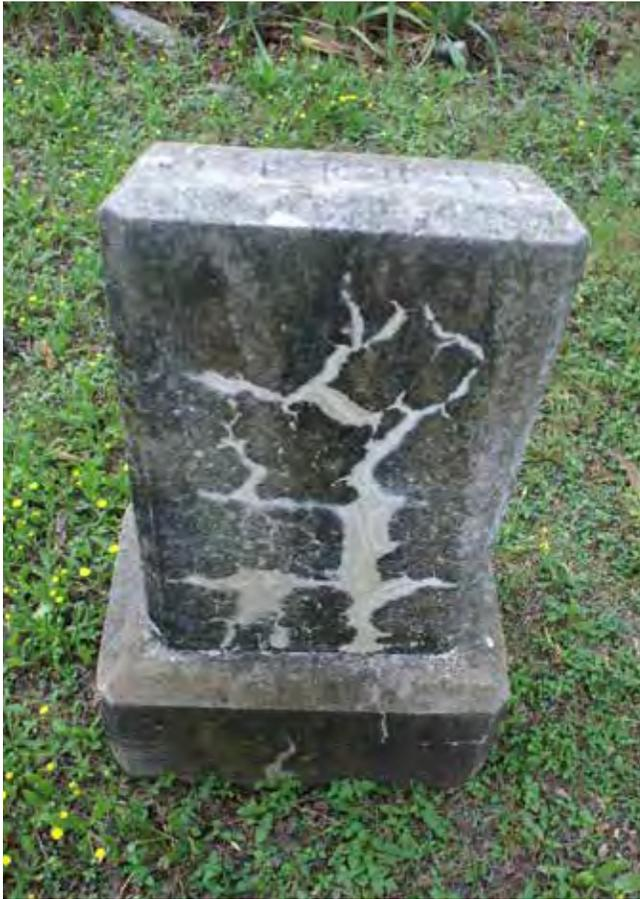
Figure 327. Repaired cracks (McDoux Preservation)
