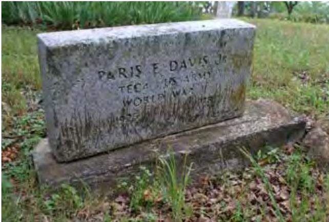
Figure 325. Marker displaced by contact with a mower and severely damaged by trimmers (McDoux Preservation)
