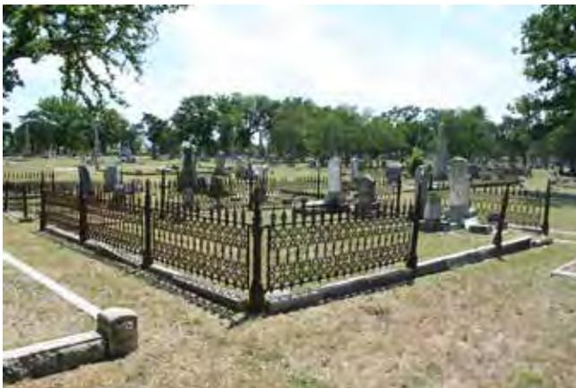
Figure 168. Cast iron fencing (John Milner Associates)
