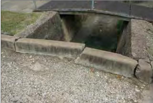
Figure 64. A severely cracked curb where the drainage channel passes beneath Main Avenue (John Milner Associates)
