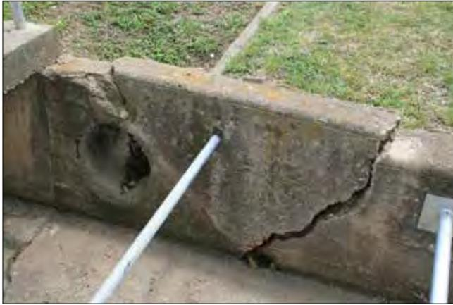
Figure 181. Partially collapsed wall section (John Milner Associates)
