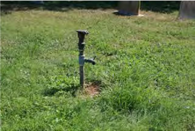
*Figure 403. A steel pipe riser, part of Evergreen's underground irrigation system (John Milner Associates)*
