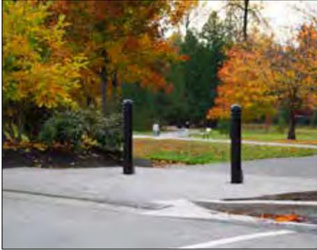
Figure 220. Removable steel bollards
