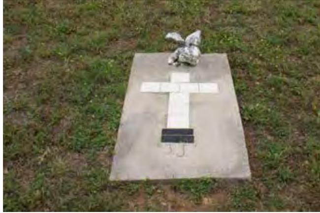
Figure 395. Concrete slab inlaid with ceramic tiles (McDoux Preservation)
