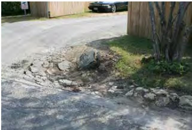
Figure 453. Damage to the road surface from turning vehicles; this has since been repaired (John Milner Associates)
