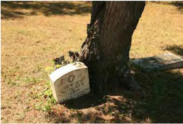
Figure 306. Tree roots causing damage to adjacent markers (John Milner Associates)
