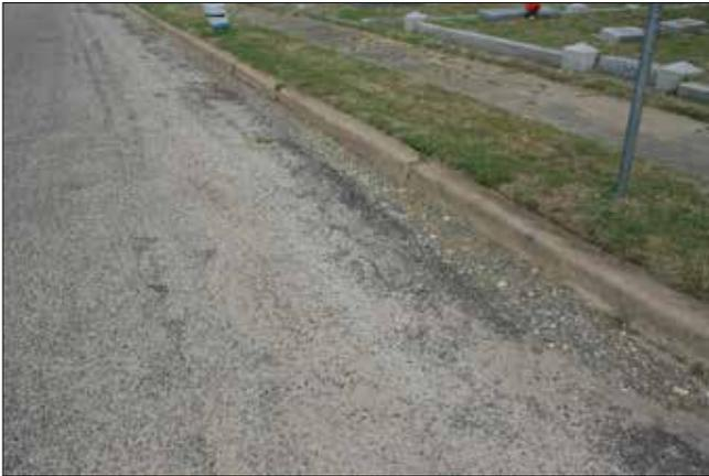
*Figure 62. Silt and gravel accumulated at the edge of Main Avenue (John Milner Associates)*
