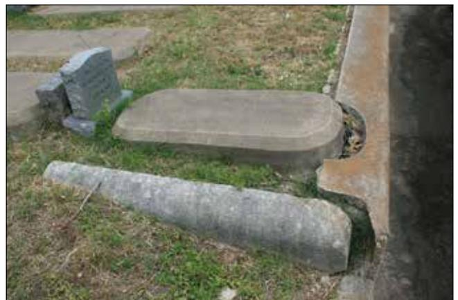
Figure 129. Markers and burials near the edge of the drainage ditch could be damaged or displaced if the walls fail. (John Milner Associates)
