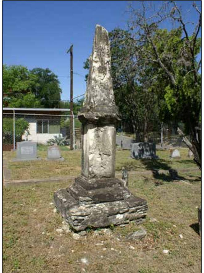
Figure 127. Severely damaged limestone monument (McDoux Preservation, OW-DSC00049)
