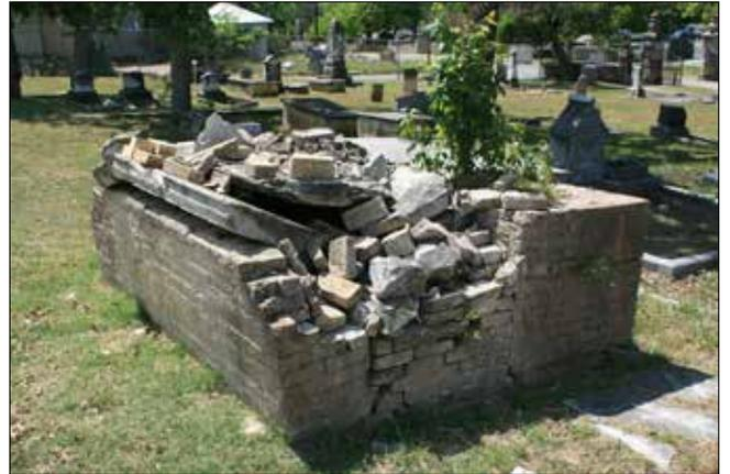
Figure 143. Deteriorated brick tomb (John Milner Associates)
