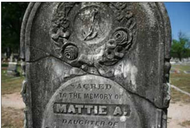
Figure 126. Previously repaired tablet marker (JMA\_050114\_0366)
