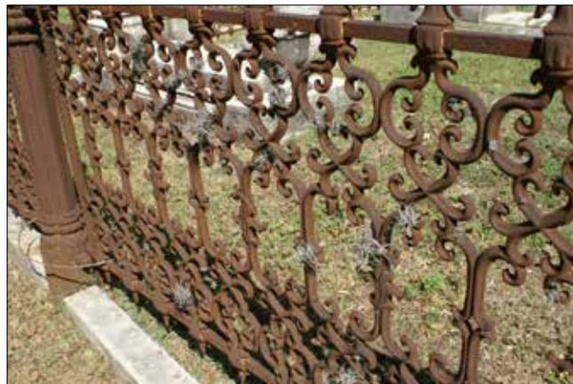
*Figure 178. Ball moss attached to rusted cast iron fence (McDoux Preservation)*
