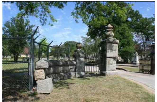
*Figure 200. Several blocks on the north wing wall of the west entrance are displaced. (John Milner Associates)*
