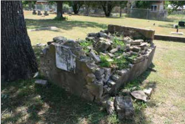
Figure 142. Deteriorated above-ground brick tomb (John Milner Associates)
