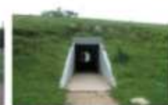
6 View of west entry of the existing pedestrian tunnel
