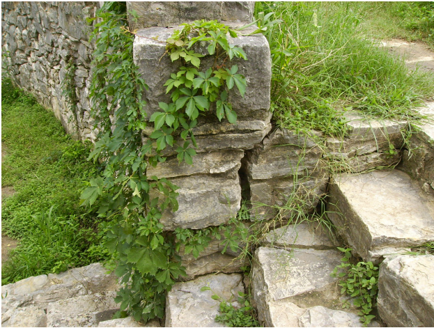
Photo 8: Inside wall of a typical stair.
