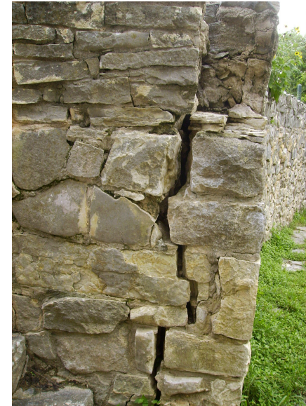
Photo 9: Inside wall of a typical stair.
