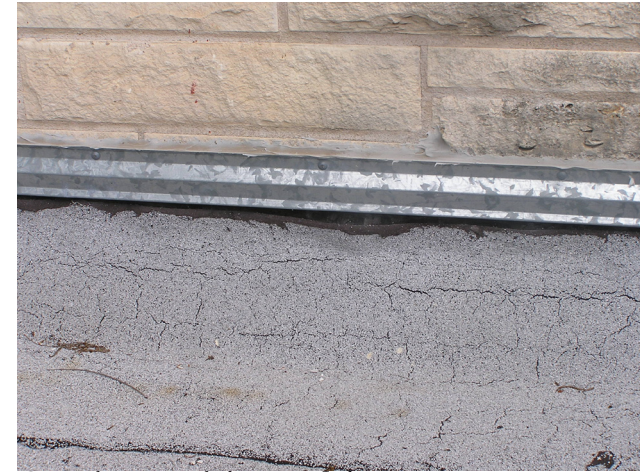
Certain locations include counter flashings at rise walls. Those metal flashings are voided in several locations.
