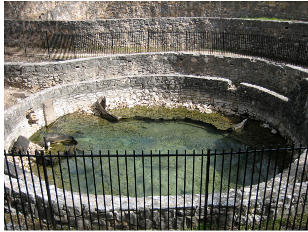
One short-term goal is to repair the walls of the spring vessel. In the same effort, add an operable sluice gate and remove sediment.
