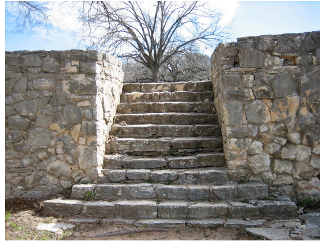
Stone stairs are in disrepair (above and right). Steps should be rehabilitated to improve footing, handrails should be added.
