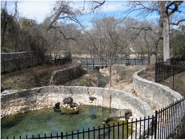
Sunken Garden in 2007. Some walls have collapsed, and the landscape is less organized. The fence is to protect the salamander habitat.
