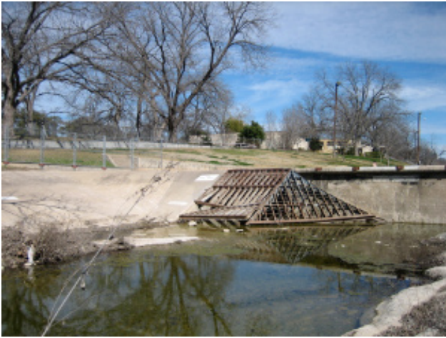
Existing inlet grate is damaged and clogs too easily.
