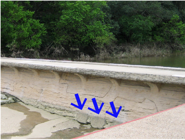
The upstream dam was built in the late 1920s with three openings in it for creek flow. These openings were closed during the 1975 construction of the bypass tunnel. One concept being considered is to install operable openings in the upstream dam.
