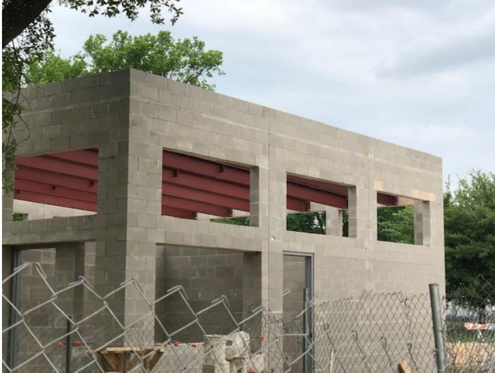
View of pool bathhouse looking east nearing completion
