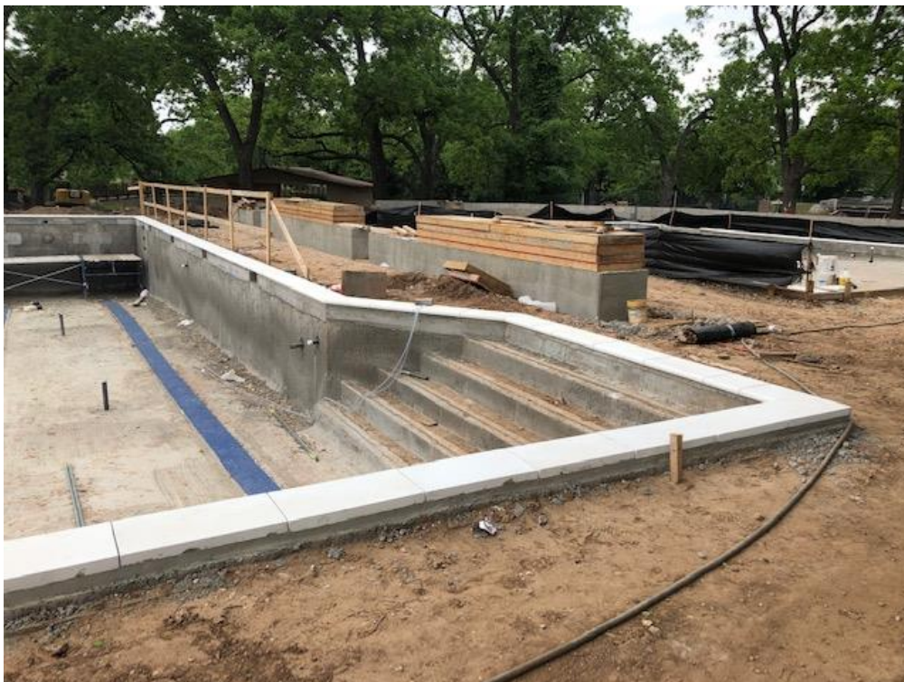
Recreational pool with coping installed
