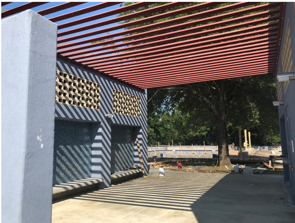
View of courtyard between the pool bathhouse and mechanical room looking towards the lap pool.
