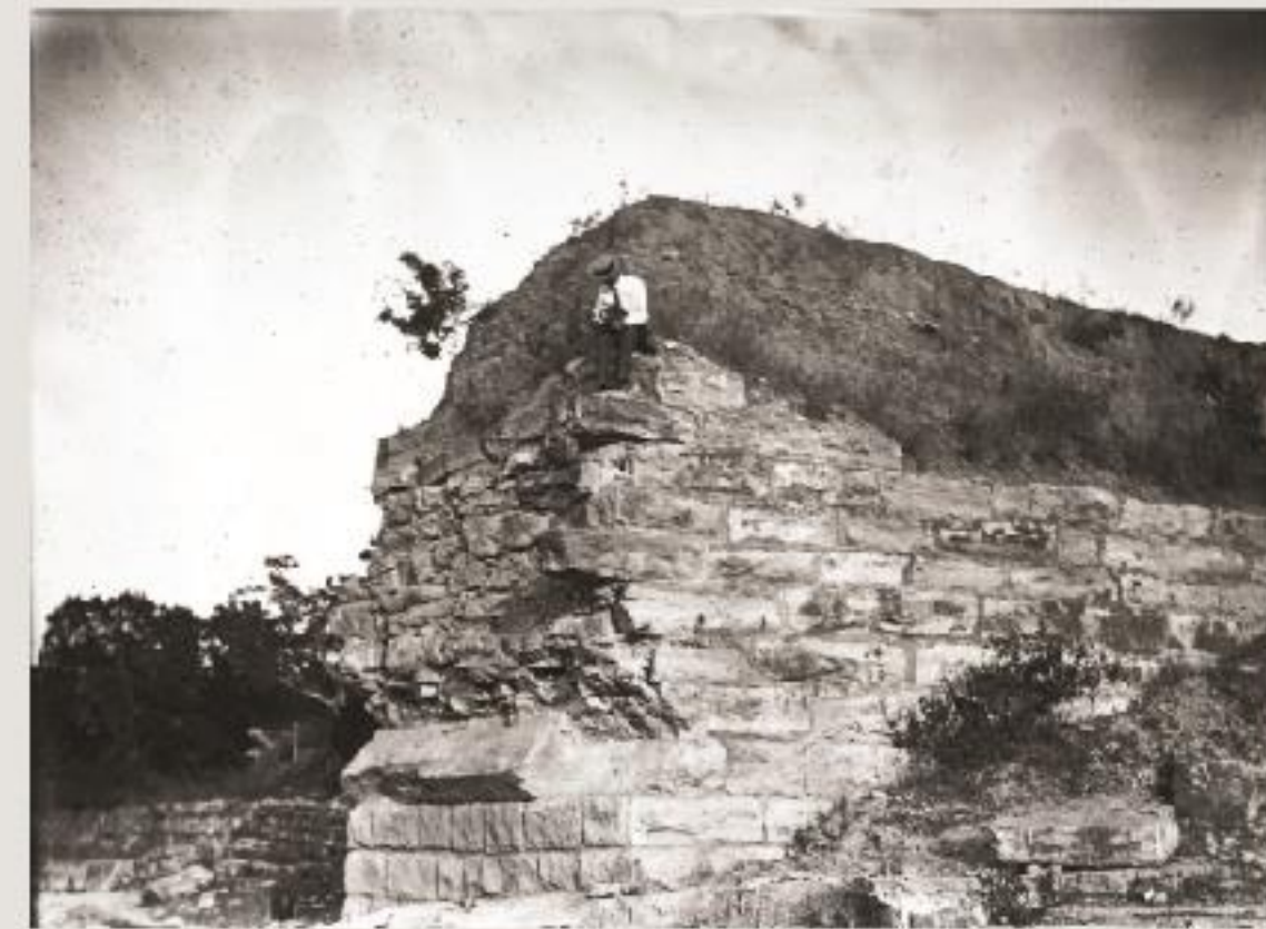
After the Flood
