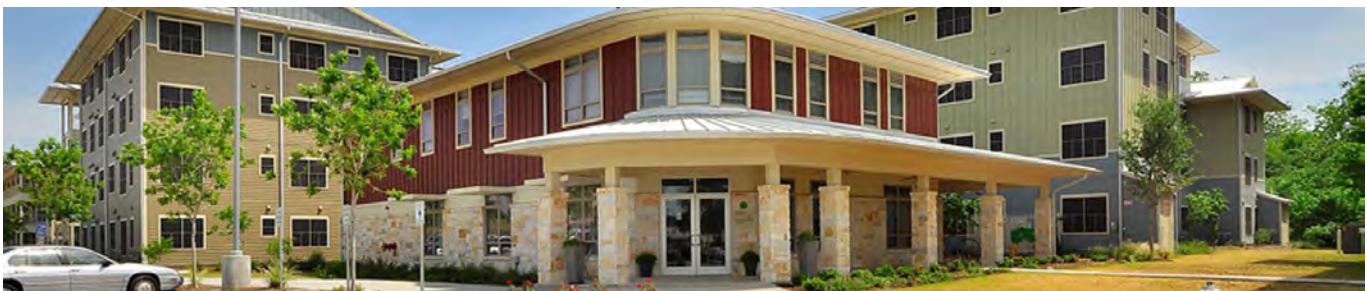
Low-income housing, M1 Station Apartments
