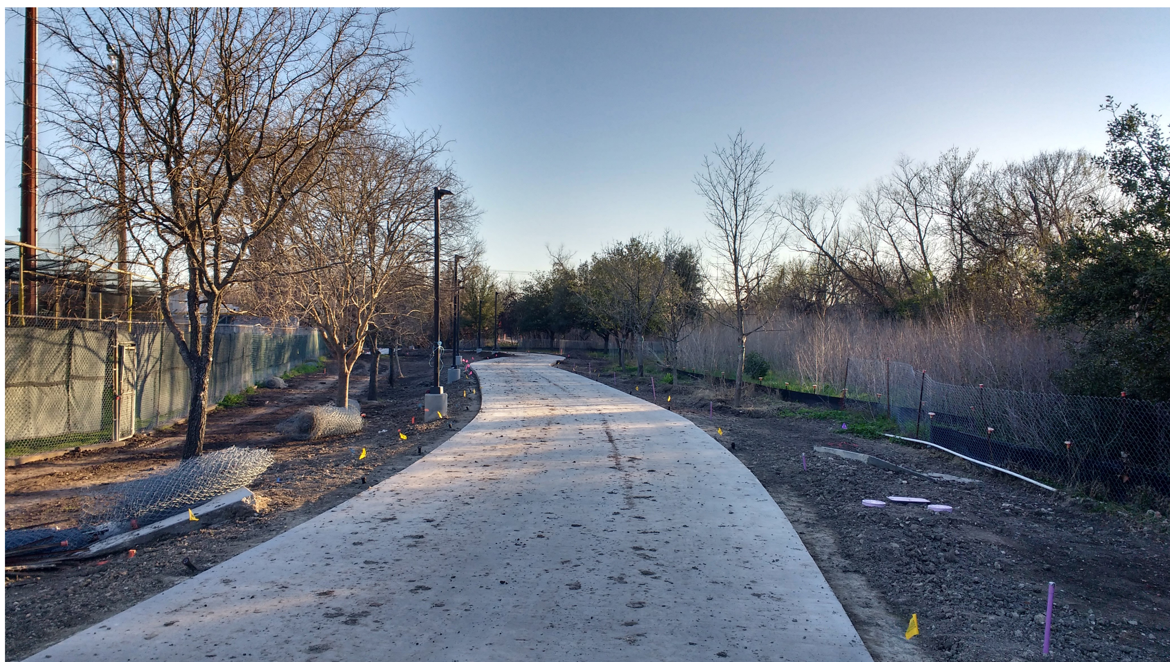
UPPER BOGGY CREEK TRAIL (UNDER CONSTRUCTION)
