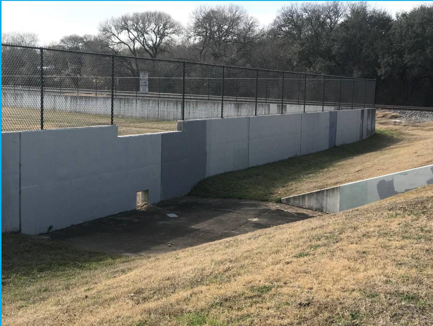
Dittmar Boulevard and Davis Oak Trail – storm water retaining walls
