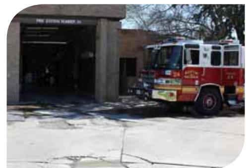
Fire station driveway replacements
