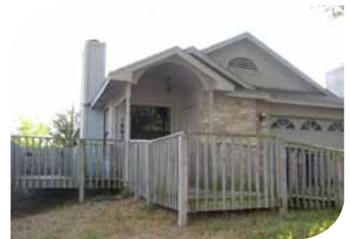
Home repair – accessibility modifications
