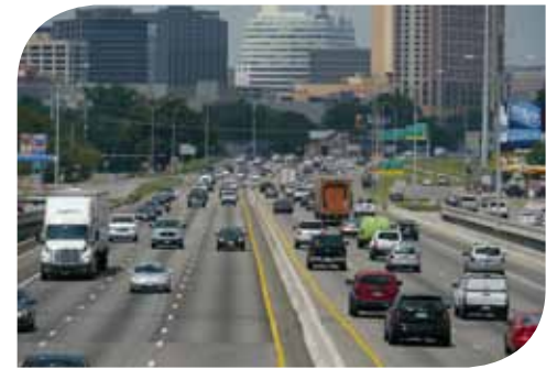
Interstate Highway 35 (IH-35)
