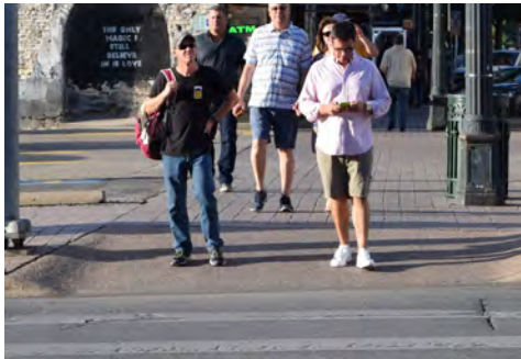
Curb ramp-slope exceeding 8.3%
