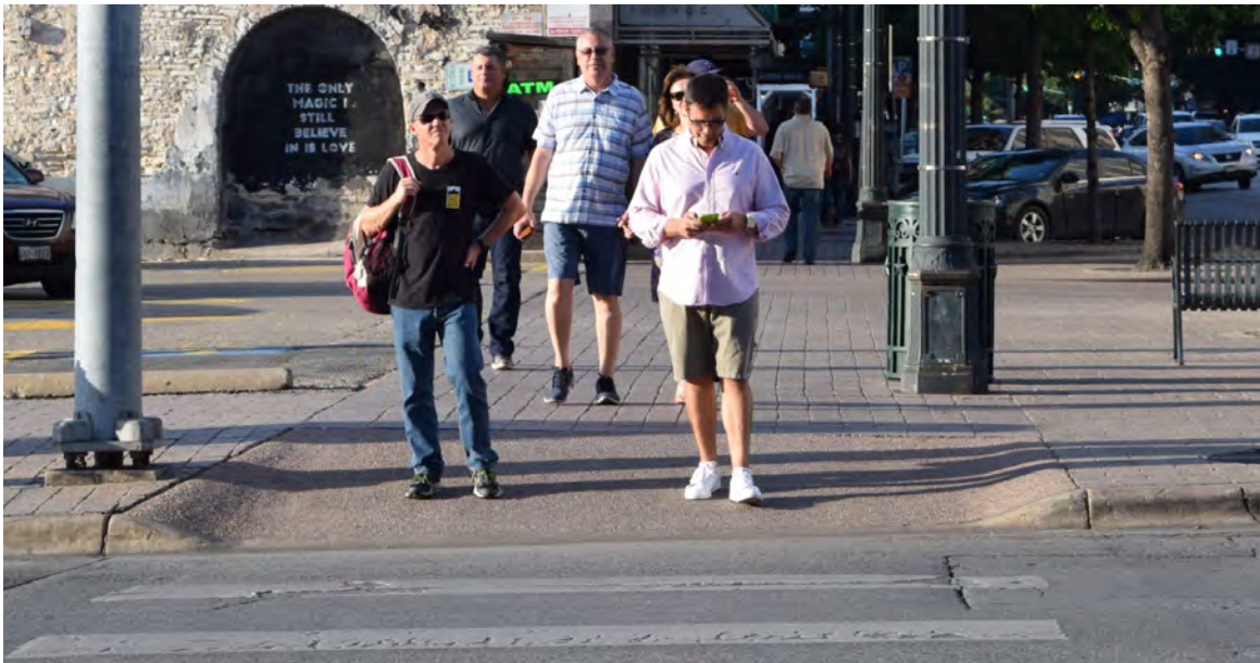
Curb ramp slope exceeding 8.3%
