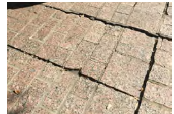
Paving in poor condition
