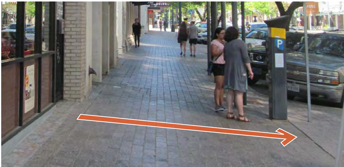
Cross-slope exceeding 2%
