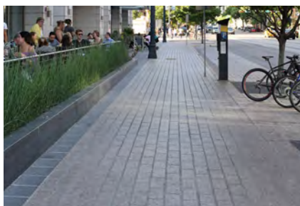
Sidewalk recently renovated - Granite pavers with contrasting darker granite border
