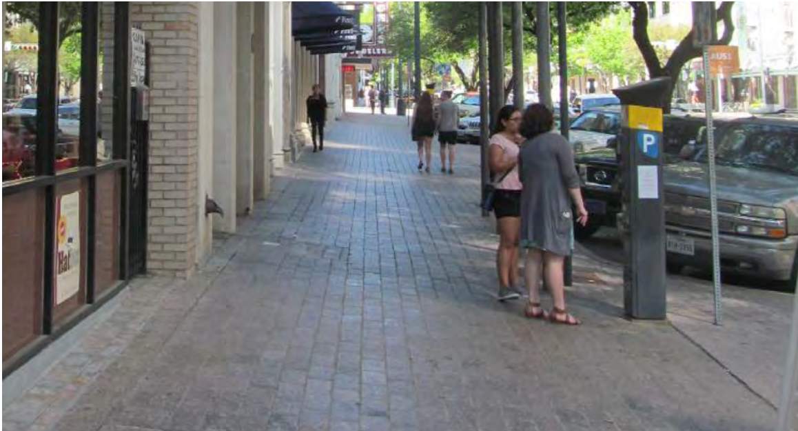
Cross-slope exceeding 2%
