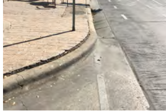
Paving in poor condition
