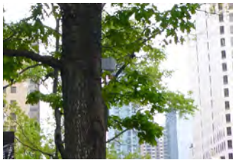
Electrical outlet embedded in tree
