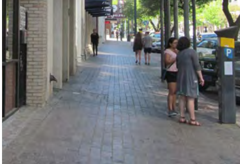
Cross-slope exceeding 2%
