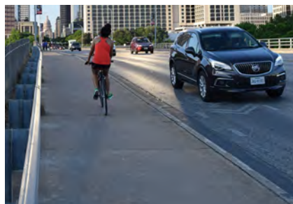
Sidewalk at bridge - Concrete
