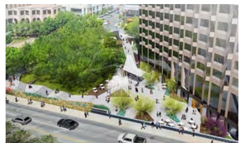
New Fareground Plaza under construction
