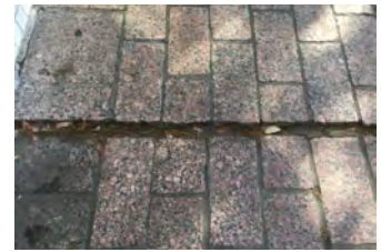
Cracked Paving
