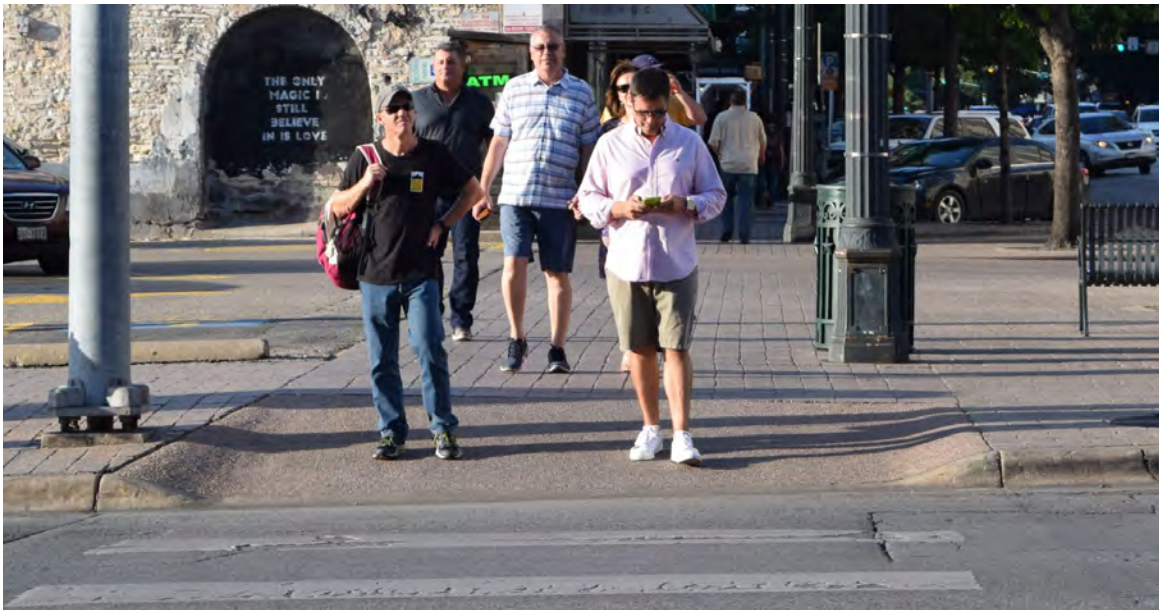
Curb ramp slope exceeding 8.3%
