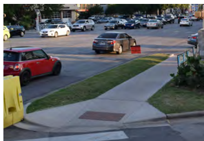
Sidewalk south of bridge - Concrete
