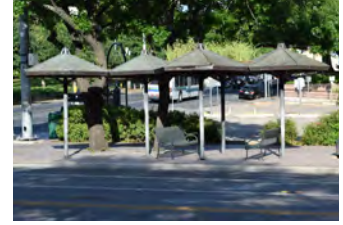
Bus stop awning
