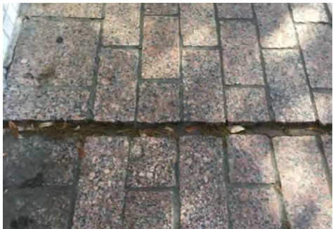
Horizontal opening exceeds 1/2"
