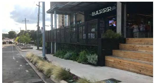
Corner of Congress Ave & Barton Springs Rd Yeti Building - Retail Space
