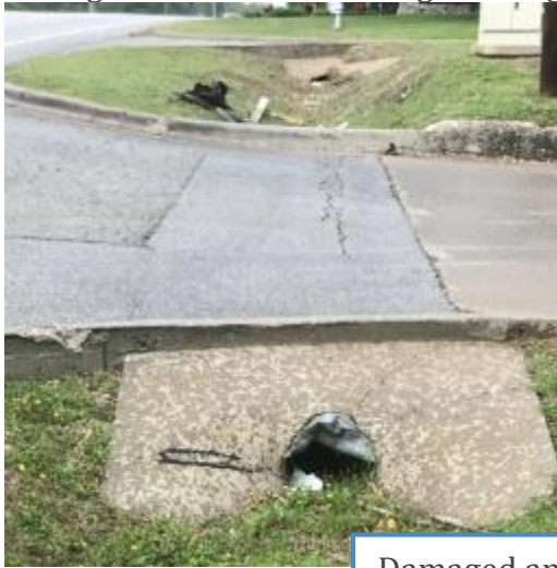
Damaged and clogged driveway culverts.
