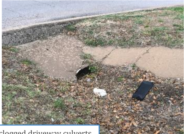
Damaged and clogged driveway culverts.
