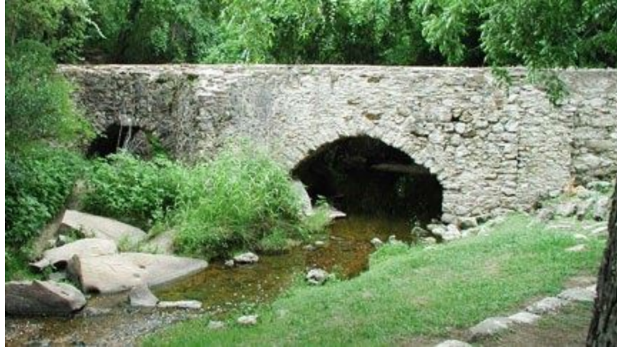
The Espada Aqueduct, Photo by Jane Thurmond, The Historic Bridge Foundation, 2003.
