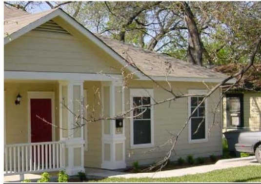
This lot was graded so a flat sidewalk could connect driveway and front door with a no-step entrance instead of a ramp.
