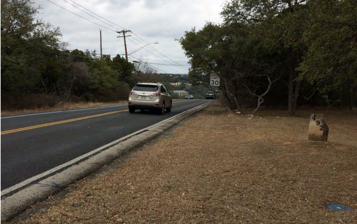
Figure 4-3 Spicewood Springs Road Picture Looking west from the top of the steep hill near 4926 Spicewood Springs Road
