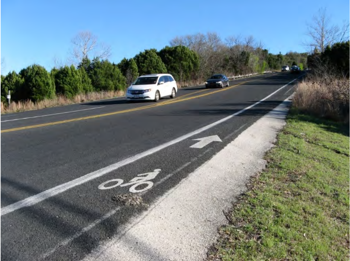
Figure 4-1 Spicewood Springs Road Picture Looking uphill from the intersection with Old Spicewood Springs Road
