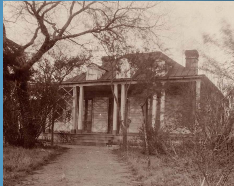
Source: Hardy-Heck-Moore, Inc. (2016). City of Austin Historic Resources Survey (Vol.2, Fig. ii-8)
