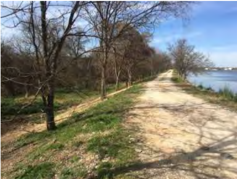
Area 2 February 2018 During Clearing
