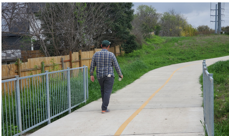
The segment of the Country Club Creek Trail connector from Burleson Rd to Ventura Dr was constructed in 2019.
