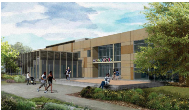
On the horizon for 2020 is the opening of the new Montopolis Recreation Center. The existing center was demolished and is being rebuilt to include facilities such as locker rooms, a gym and weightroom, and other multi-purpose rooms.
