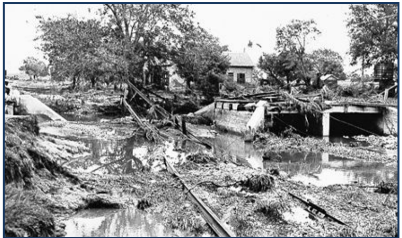
Damage from the 1935 Flood
