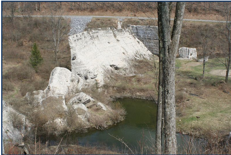
Remnants from the Austin Dam
