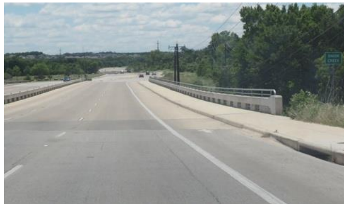
Figure 3-5: Onion Creek Bridge
