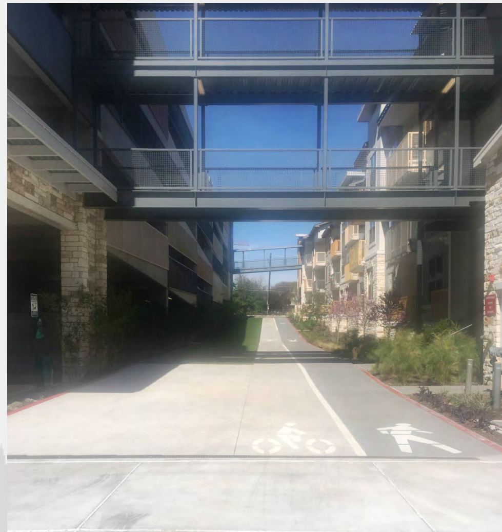
Saltillo Station, E 5th, Internal Circulation Route
