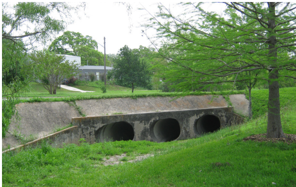
Before construction, a culvert and street bisected the park
