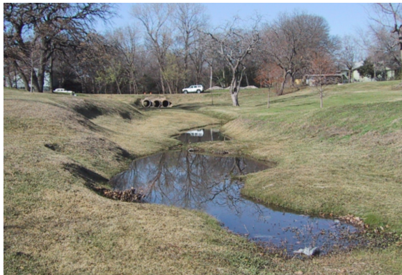
Mowed, dredged channel with turfgrass banks.
