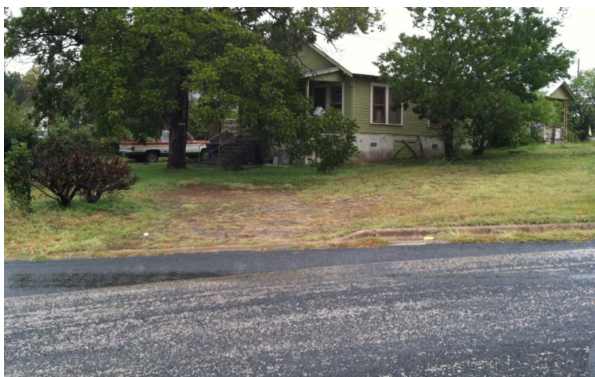
Site of rain garden at Denver Avenue on City of Austin property before construction
