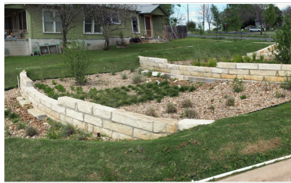
The rain garden captures and cleans storm water from the adjacent road and the bike/pedestrian trail
