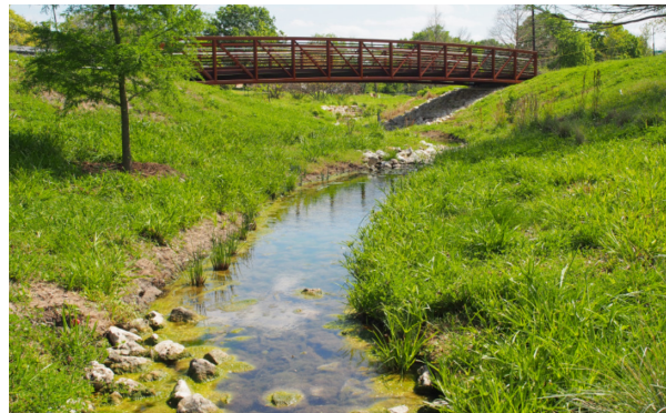
A bike/pedestrian bridge replaced the culvert and hydrologically reconnected the stream
