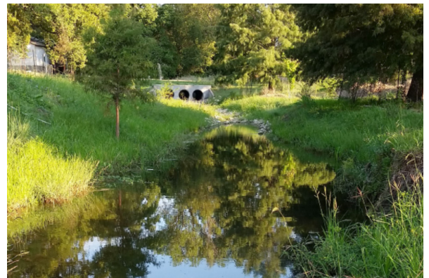
Restructured channel with riffle/pool complex and native riparian vegetation.
