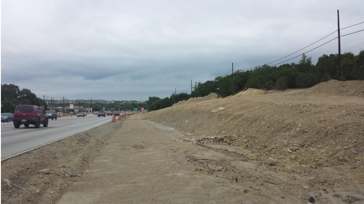
Figure 22 - US 290 Eastbound near intersection with SH 71 5-13-14. No temporary stabilization, no controls.
