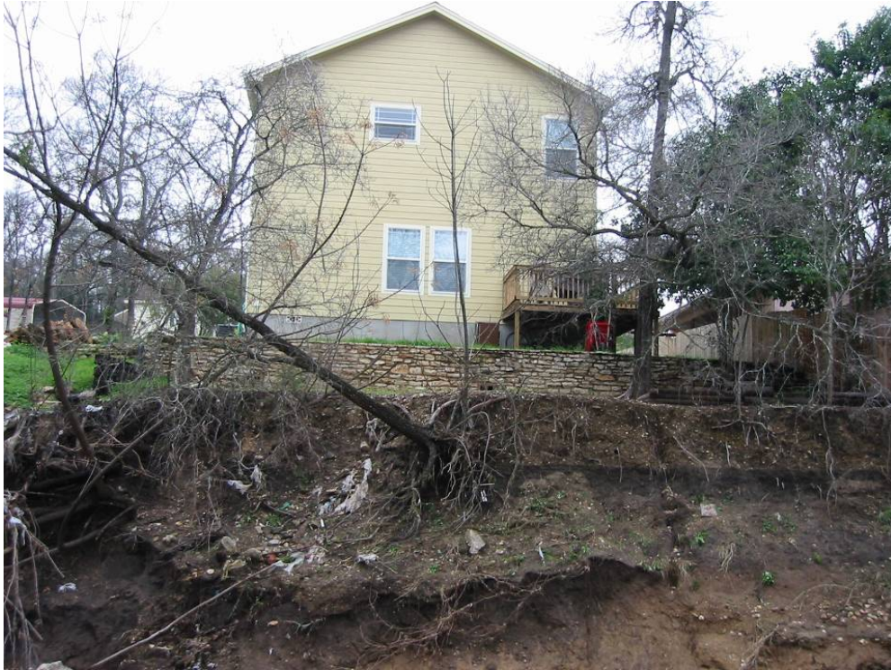
House Built within an Erosion Hazard Zone
