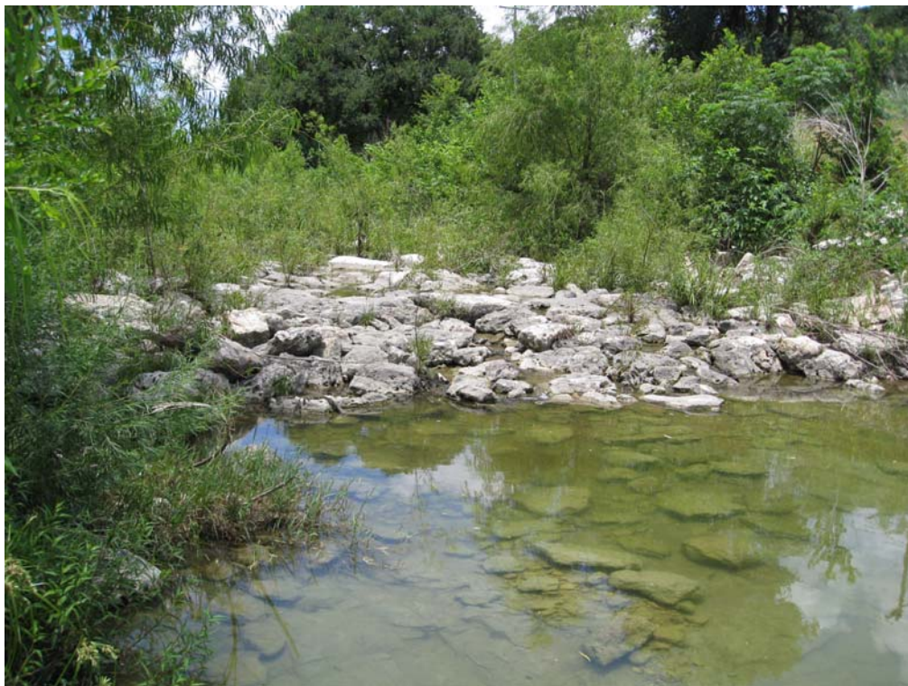
Example Rock Grade Control Structure
