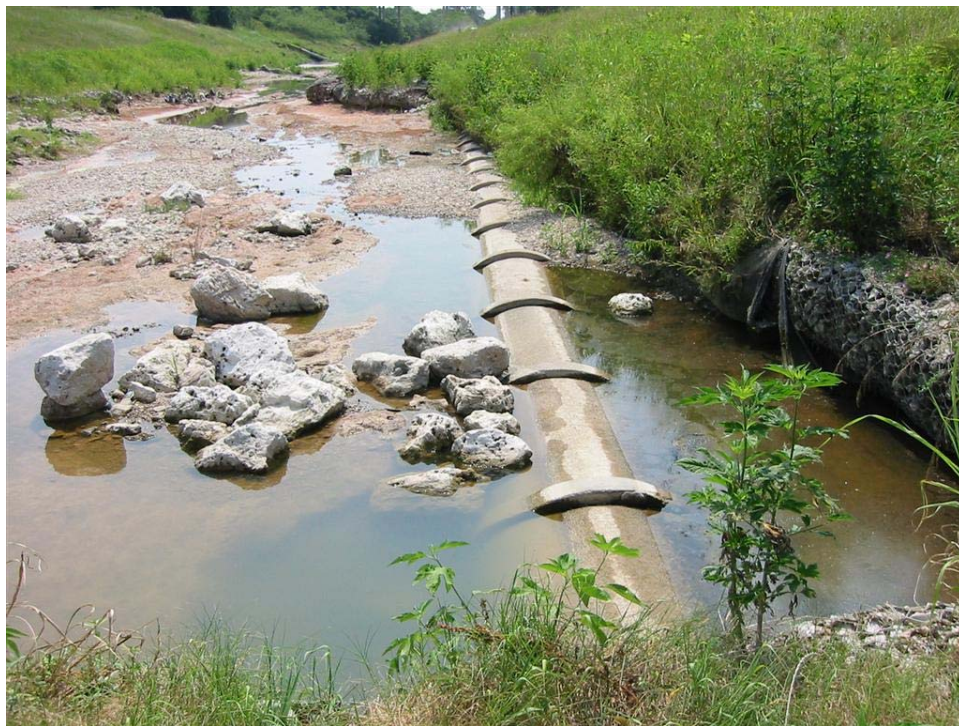
Exposed Utility within an Erosion Hazard Zone
