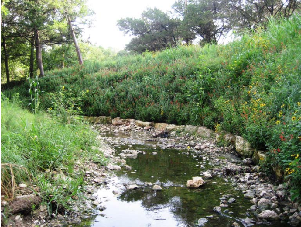
Example Bioengineering Bank Stabilization
