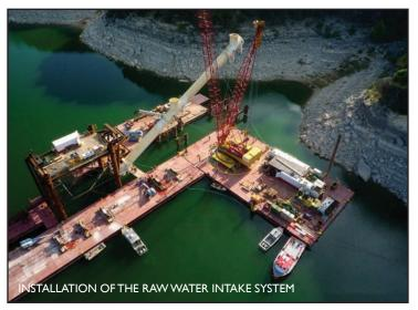
The intake system consists of three stainless steel screened inlets, each of which is installed at a different depth. Only one screen will be used at any given time to draw raw water from the Lake. Which screen is used will depend on the current lake level to optimize raw water quality, which in turn helps increase treatment efficiency.
